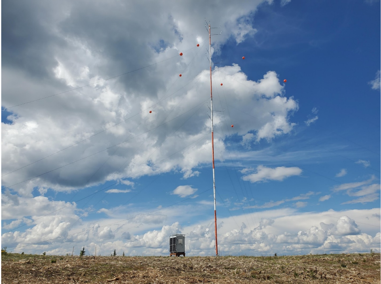
Example of an existing meteorological tower currently installed on the project site.
