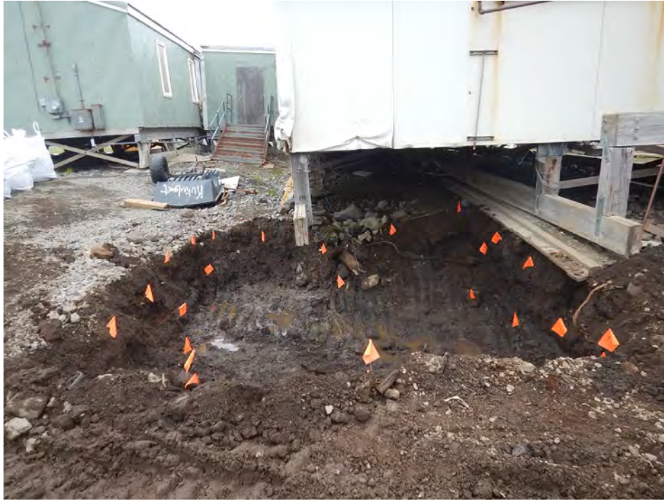
Photograph 9: Field screening pin flag grid in excavation, view northwest.
