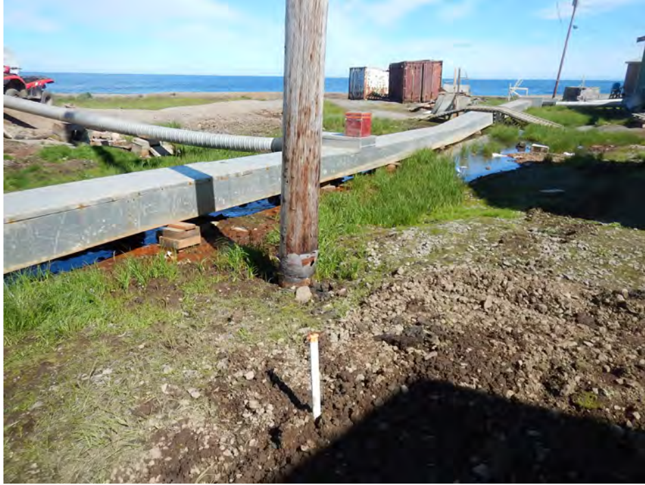
Photograph 17: WP-05 on north side of building, view northeast.
