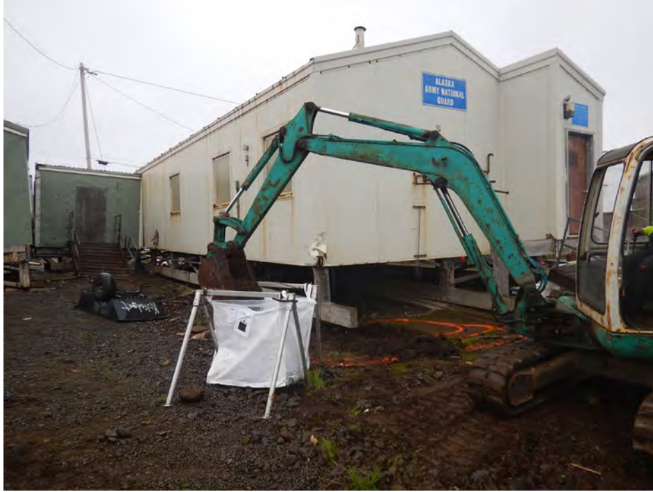
Photograph 3: Beginning excavation, view north.
