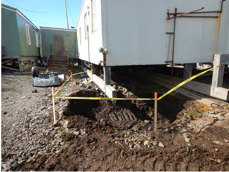
Photograph 5: Excavation at 12 cubic yards removed and 3 feet deep, view north.
