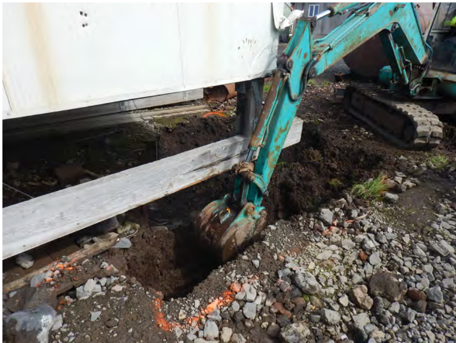
Photograph 4: Excavation at 10 cubic yards removed, view east.
