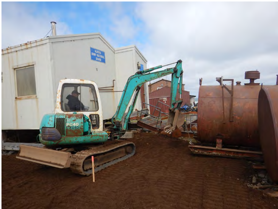
Photograph 12: Pulling ASTs back into position, view north.
