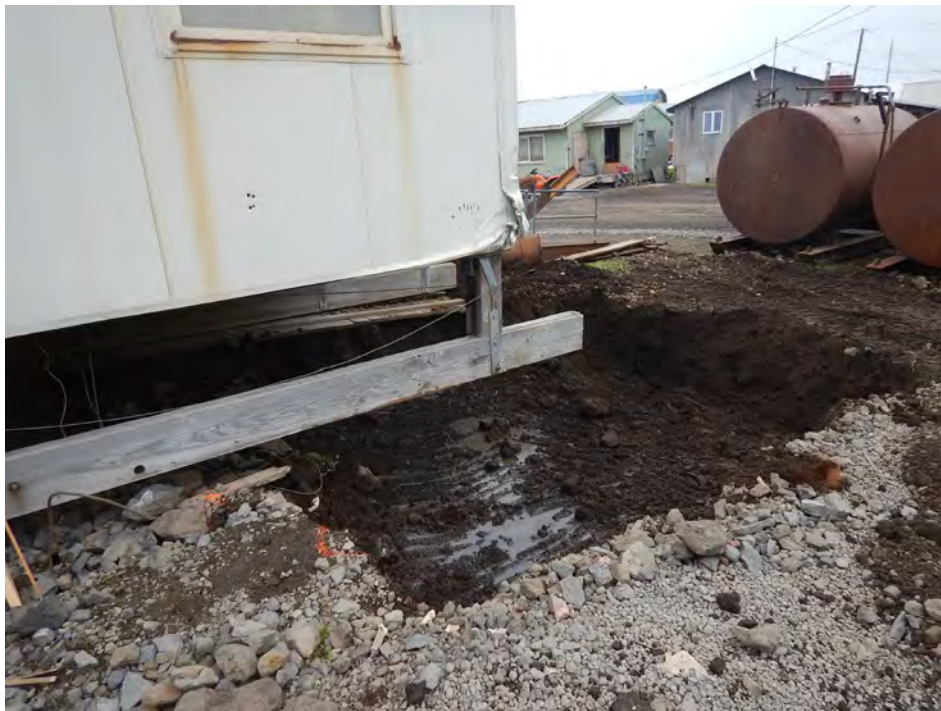
Photograph 8: Completed excavation at 30 cubic yards removed, view east.
