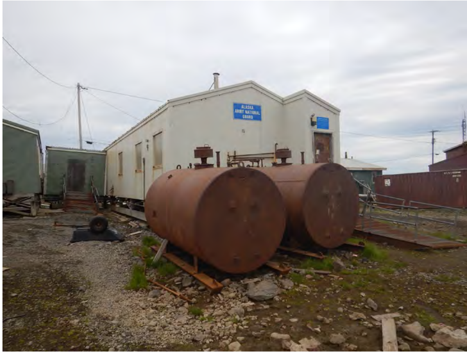
Photograph 1: FSA buildings and ASTs, view north.
