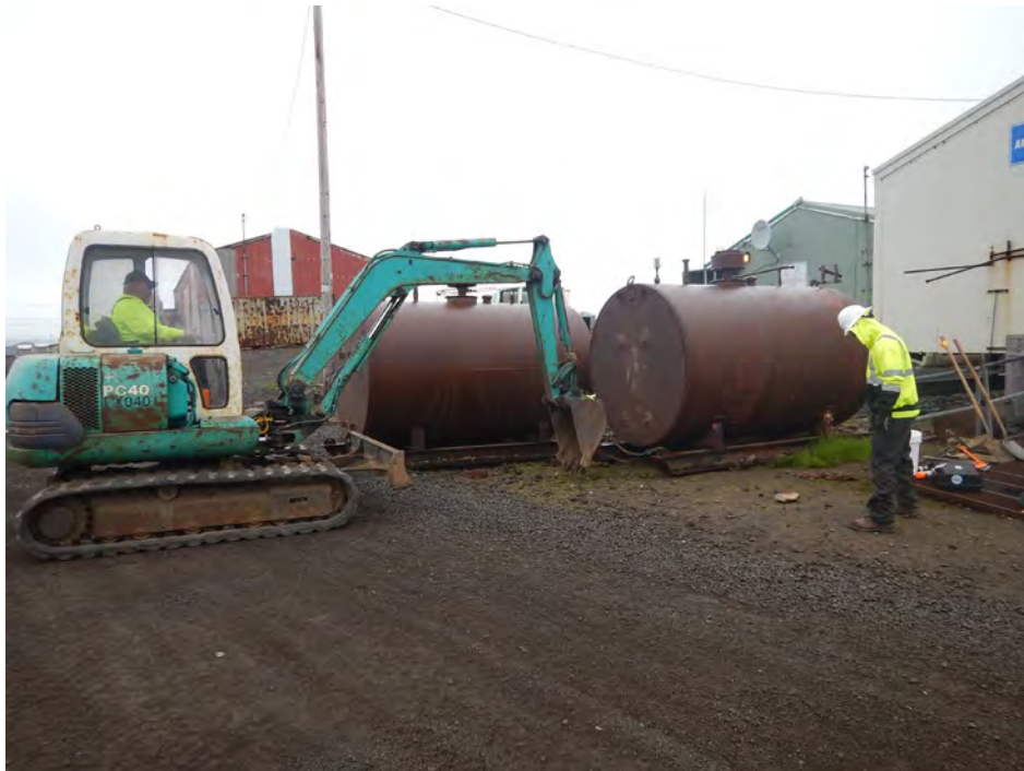
Photograph 2: Moving ASTs to southwest for removal action, view west.
