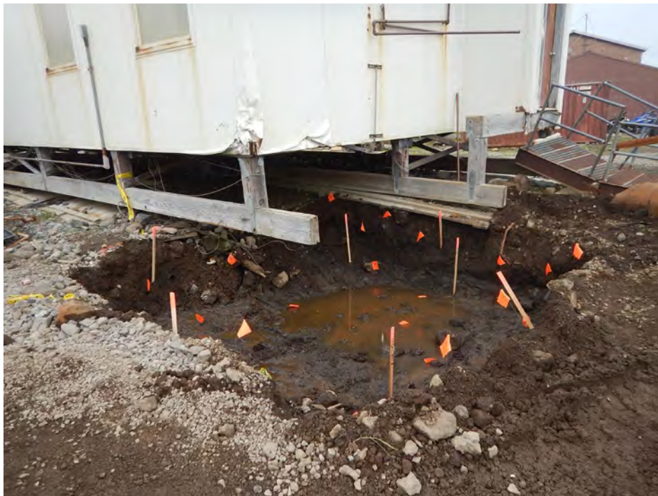
Photograph 10: Sample locations marked with stakes in excavation, view north.
