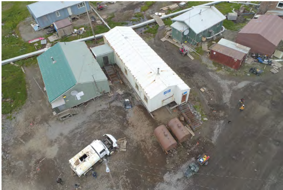
Photograph 20: Aerial view of FSA following site restoration, view northeast.
