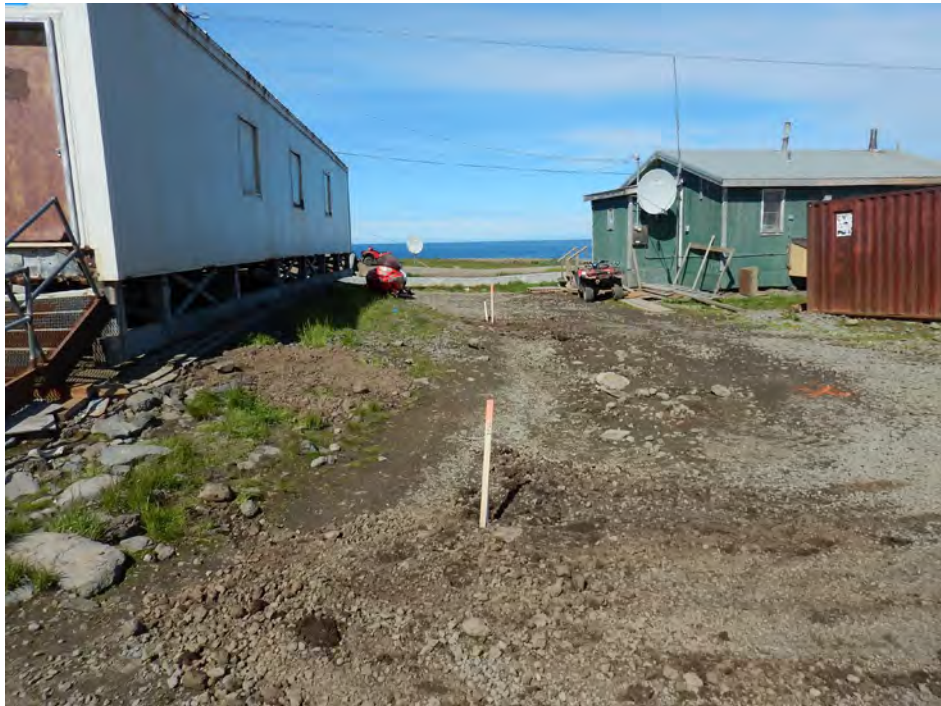
Photograph 16: WP-03 and WP-04 as seen from road on east side of FSA, view northeast.
