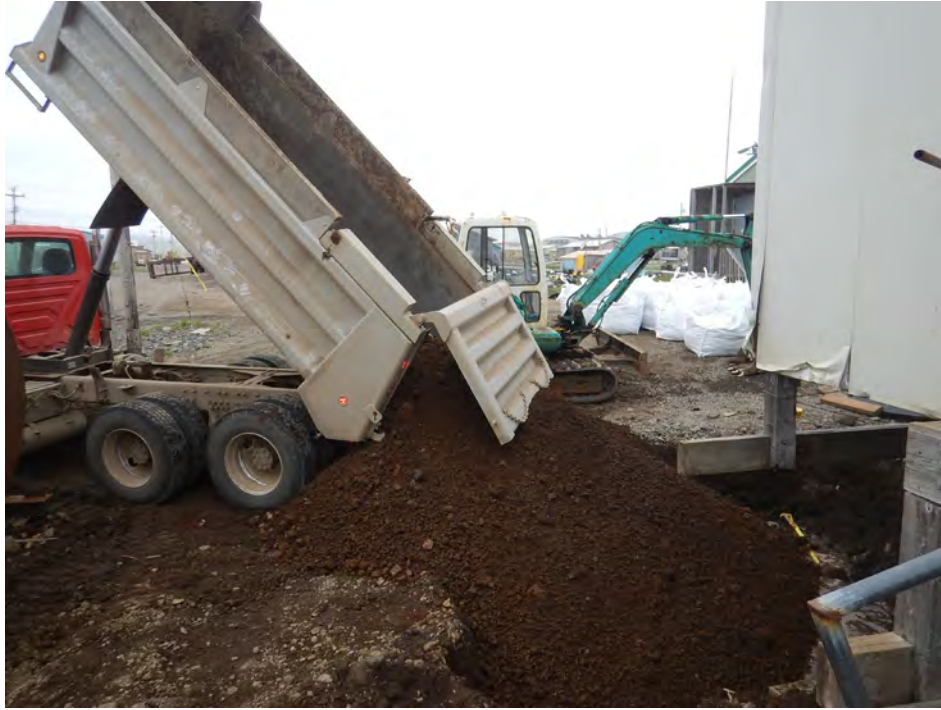
Photograph 11: Backfilling excavation, view south.
