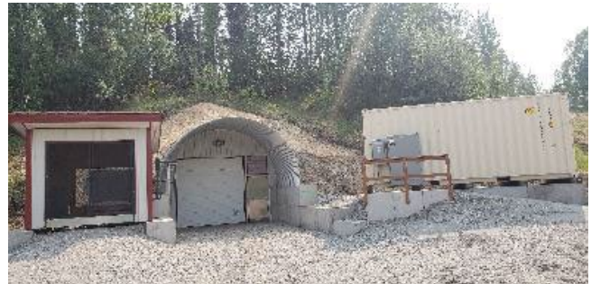
Figure 3. Permafrost Tunnel Entrance.
