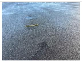
Section 04 of the apron was initially constructed in 2004 and has had no major work since. The most common distresses observed are low severity longitudinal and transverse cracking, large quantities of low to high severity raveling, and low severity weathering. In field observations include an increased loss of the fine aggregate which is exposing the coarse aggregate and in some areas the removal of the coarse aggregate altogether.
