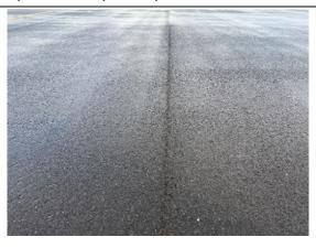
Sections 02 and 03 of the aprons were initially constructed in 1981 while section 01 was initially constructed in 1996. All three sections' most recent major work was a mill and overlay of 6" in 2014. The most common distresses observed are low severity longitudinal and transverse cracking, small quantities of low severity raveling, and low severity weathering. In field observations include the degradation of the paving joints causing longitudinal cracking and raveling to develop.
