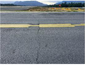
Taxiway A was initially constructed in 1981 and its most recent major work was a mill and overlay of 6" in 2014. The most common distresses observed are low severity longitudinal and transverse cracking, low severity raveling, and low severity weathering. In field observations include the degradation of the paving joints causing longitudinal cracking and raveling to develop.
