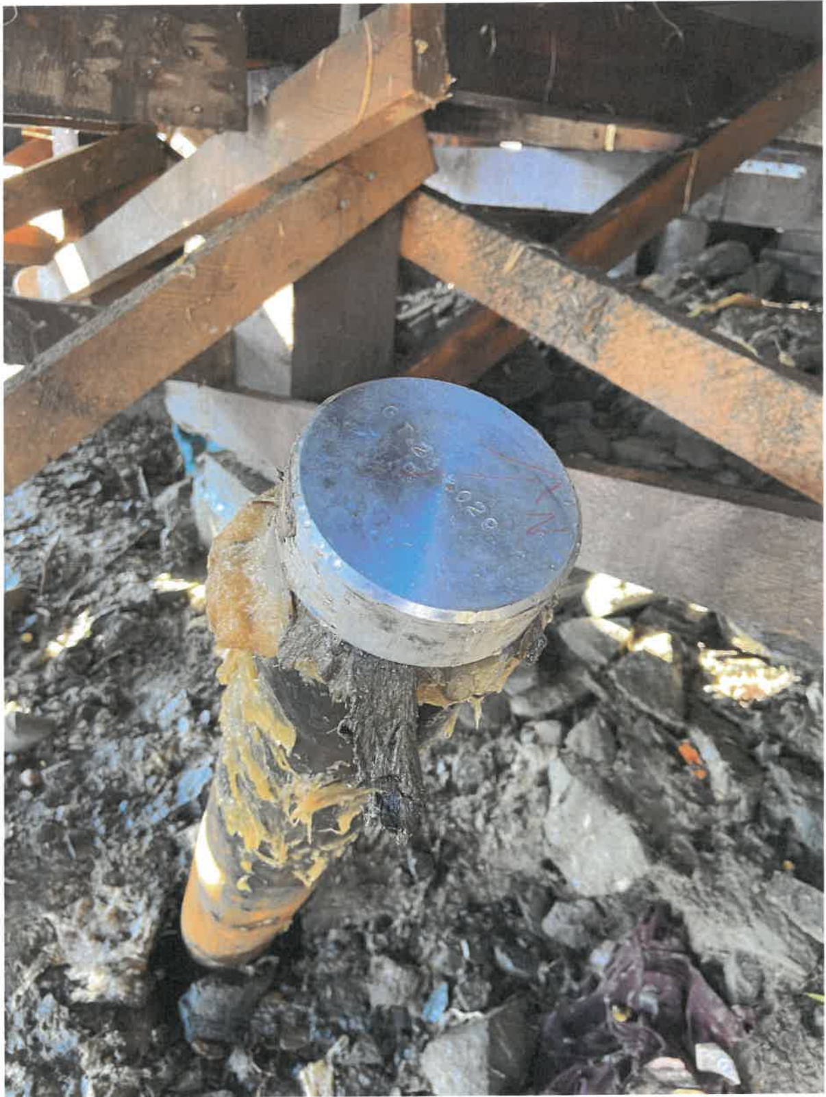
Photo 39: Stryker Pad diamond drill hole GT23-029 is capped.
