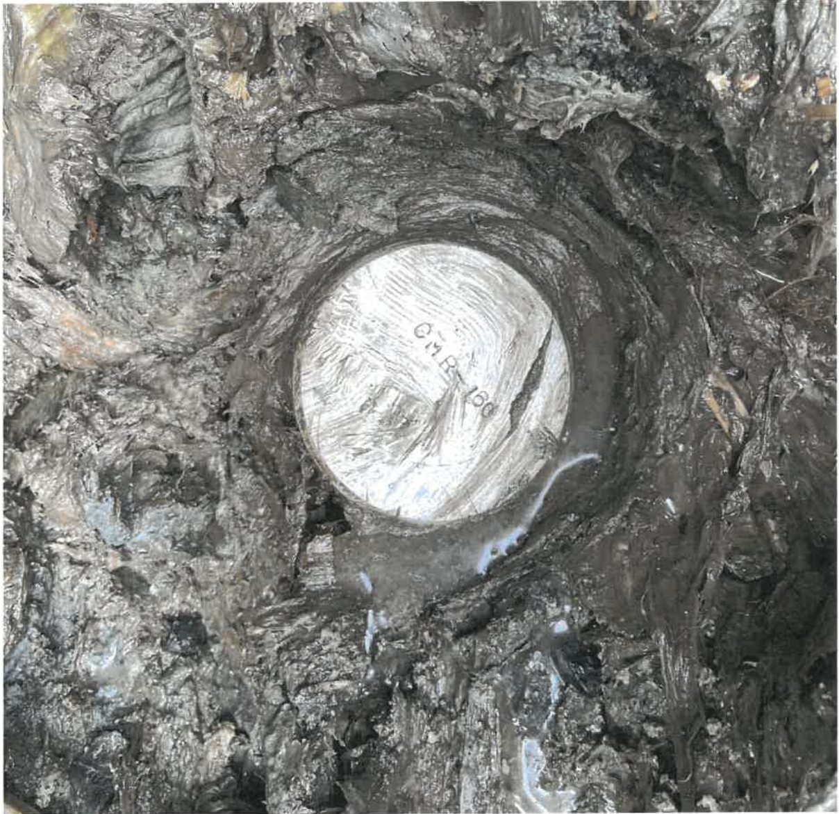
Photo 12: KD Pad diamond drill hole CMR23-160/01 is capped.
