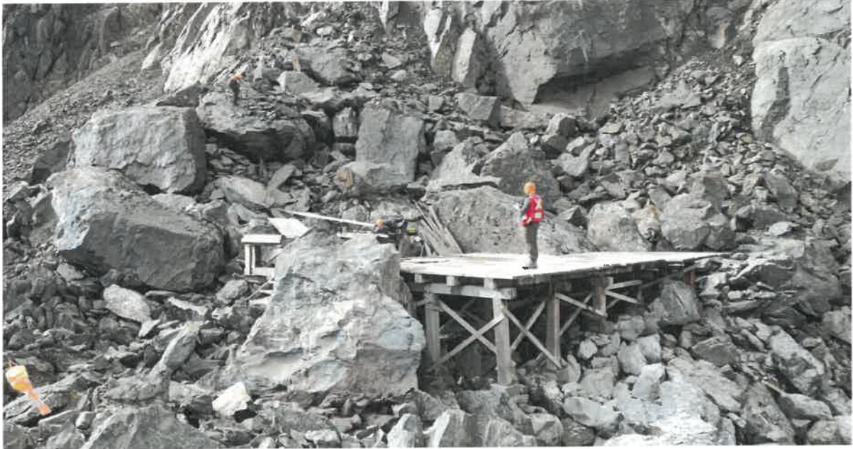
Photo 64: Merrill's Drill Pad after construction.
