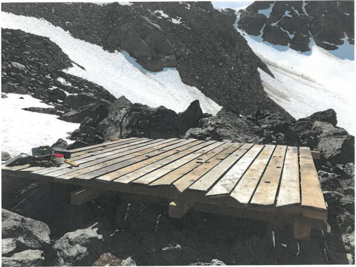
Photo 105: Mid-Station Pump pad. Pad retains decking and remains unreclaimed for future use.
