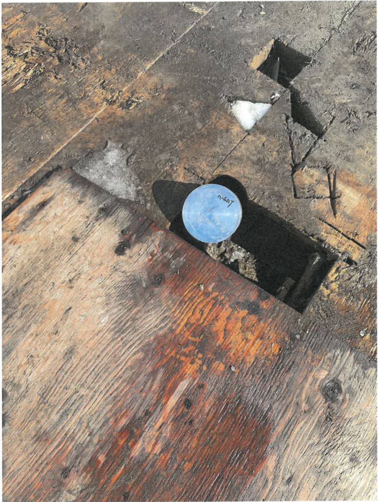
Photo 35: UM Pad diamond drill hole GT23-025 is capped.
