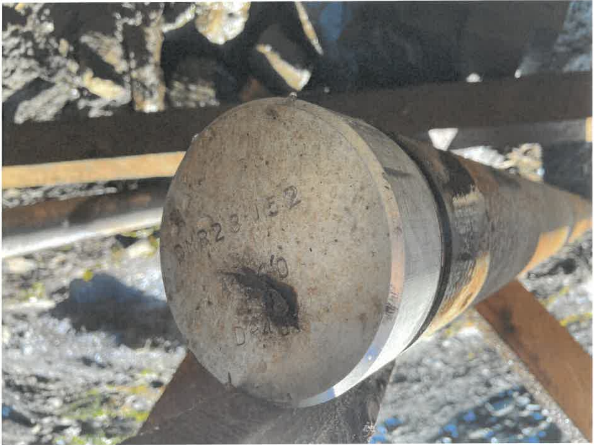
Photo 4: Stryker Pad diamond drill hole CMR23-152 is capped.
