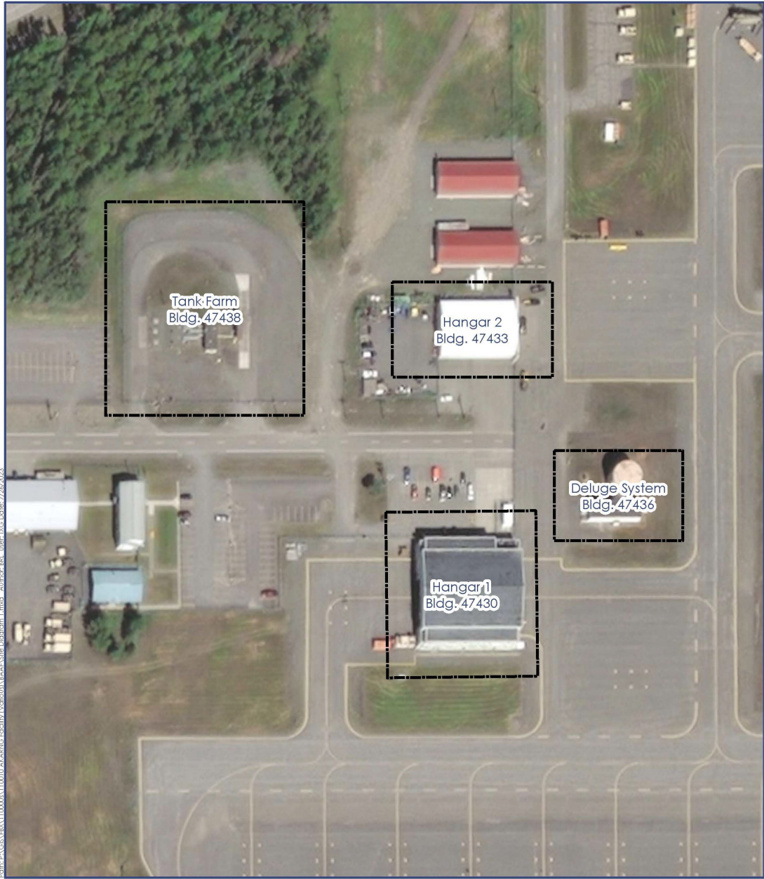
July 2023 TANK FARM, HANGARS 1 & 2, AND DELUGE SYSTEM Figure 3
