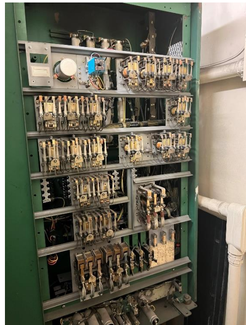
4. The existing controller is the original 1968 relay design.
