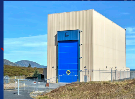
Payload Processing Facility
