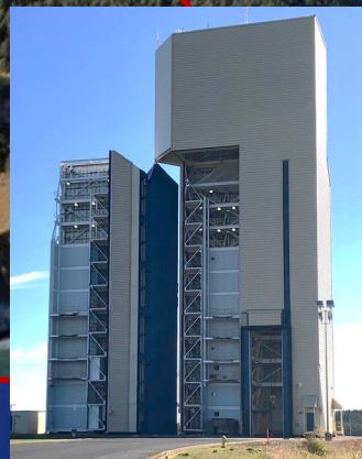
Launch Service Structure (Launch Pad 1)
