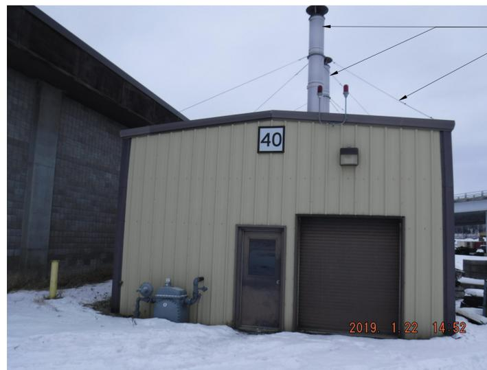
REMOVE TWO EXISTING BOILER ROOF STACKS & GUYE WIRES
