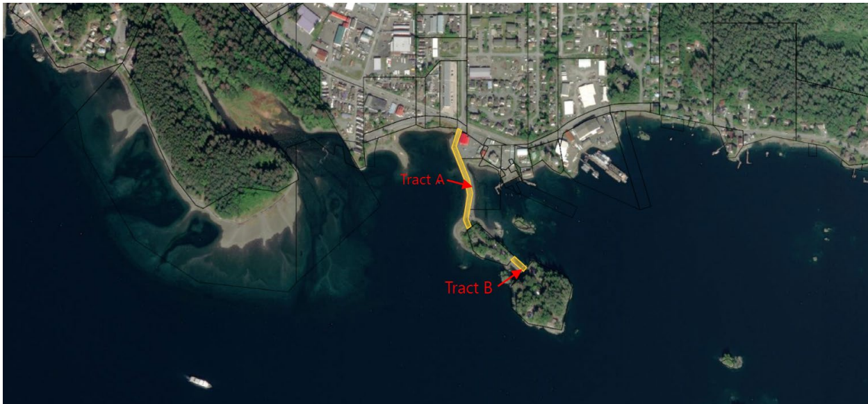
Figure 1. Aerial photo of Tract A and Tract B of the proposed easement on Raven and Cannon Island.
