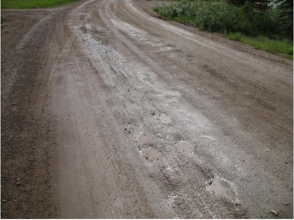
This example has a crown, sufficient compacted surface material at the shoulders but not on the crown. There are no soft spots or sinkholes and the water will drain from the shoulders, however there is some wash boarding and potholes. This road would need to be graded, gravel recovered from the ditches, the crown reshaped and the road re-compacted.
