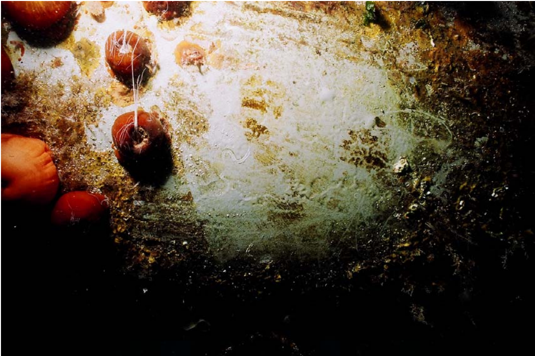
13. Hull of pontoon Note coating blisters
