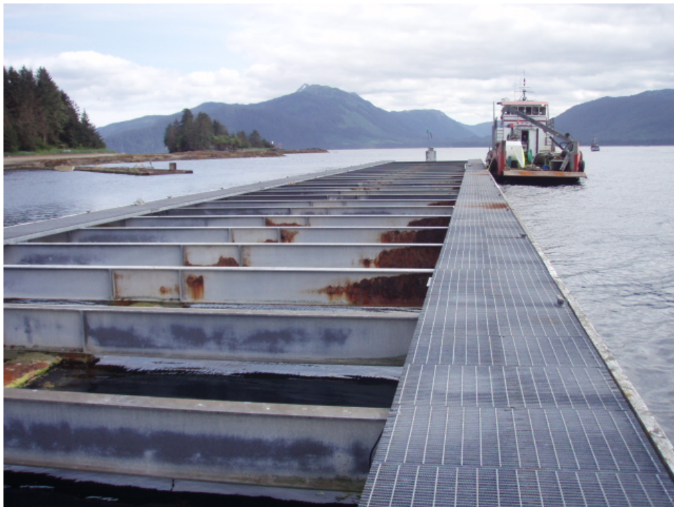
8. Steel breakwater
