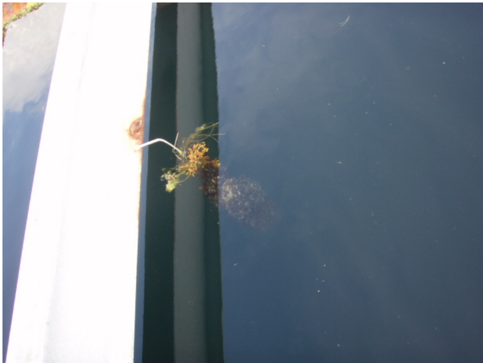
6. Hanging anode connection
