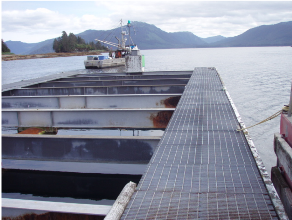
3. Steel Breakwater
