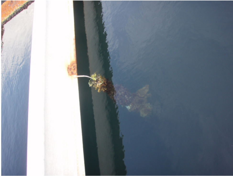
7. Hanging anode connection
