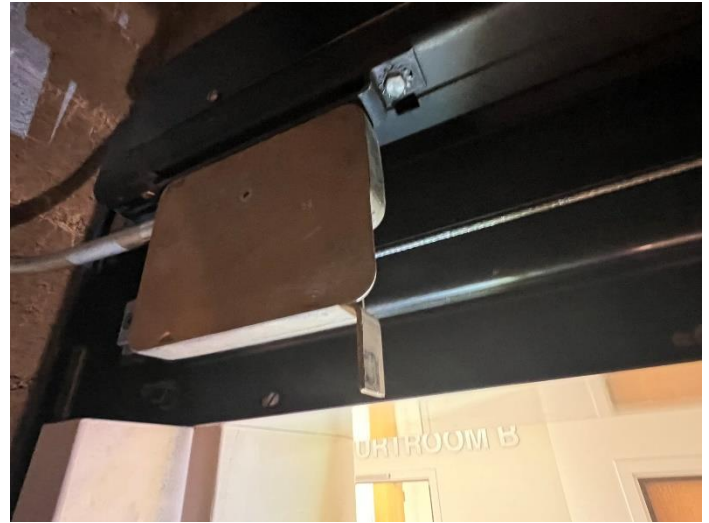
10. The interlocks will be retained. New contacts will be provided.
