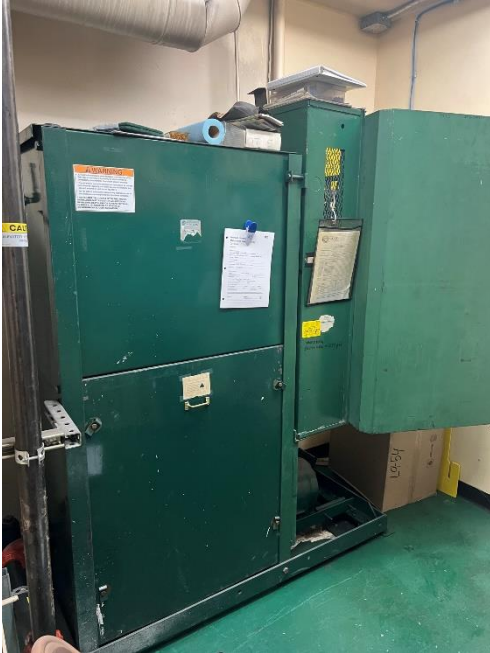
1. The existing power unit uses a dry unit design. The new power unit will use a submersible design.
