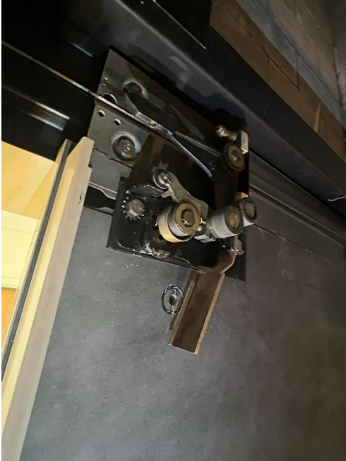
9. The car door pick up rollers can be retained/refurbished.
