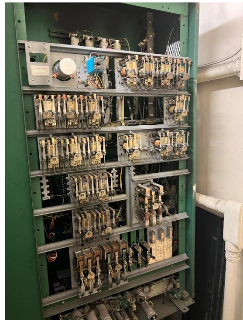
4. The existing controller is the original 1968 relay design.
