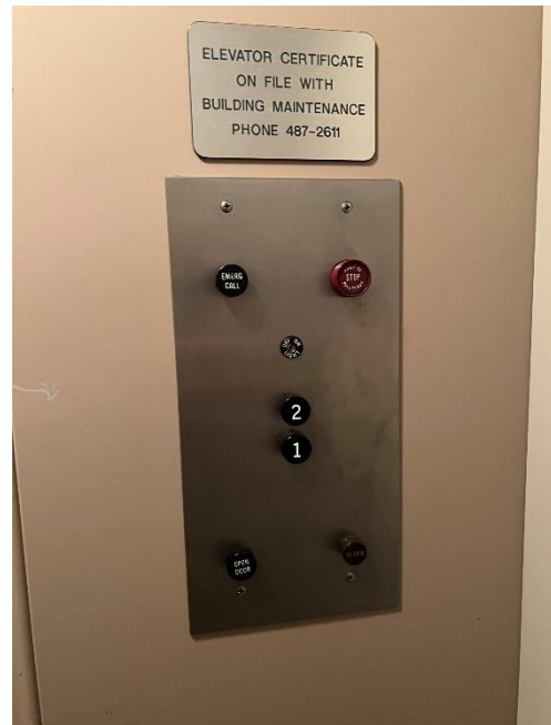
12. A new ADA compliant car operating panel will be provided.
