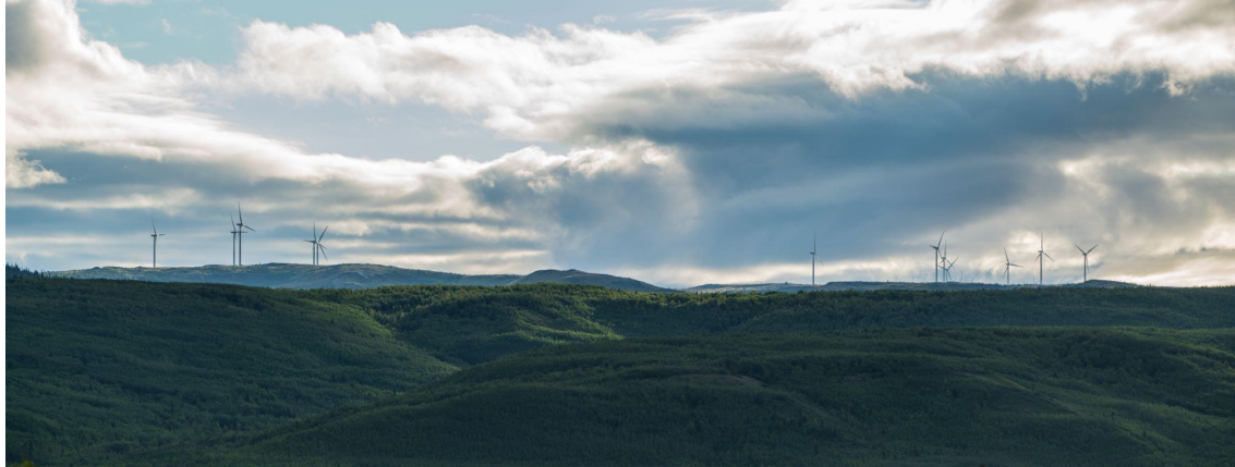
Figure 1. View of the existing Eva Creek Wind Farm (est. 2011) operated by Golden Valley Electric Association outside of Healy, AK. The proposed Shovel Creek Wind development would have many attributes in common with this existing project; however, electrical system modeling shows that this project could reliably provide >25% of GVEA's total annual energy needs with zero carbon emissions.
