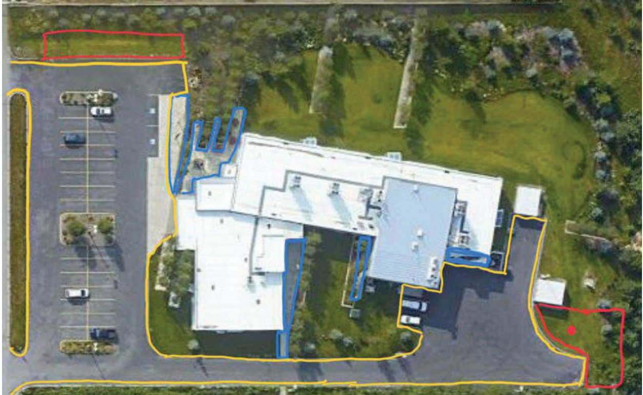
Full image of the parking lot and sidewalks
