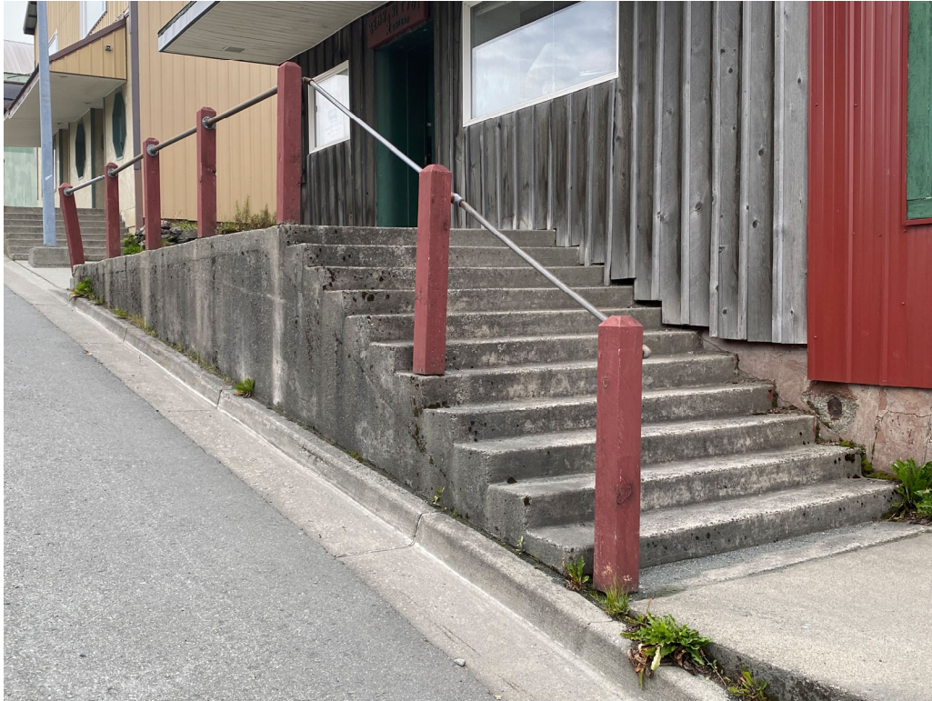
Figure 7 - Existing conditions at Pipe Hand Rail 3. Photograph dated 09/06/2022.
