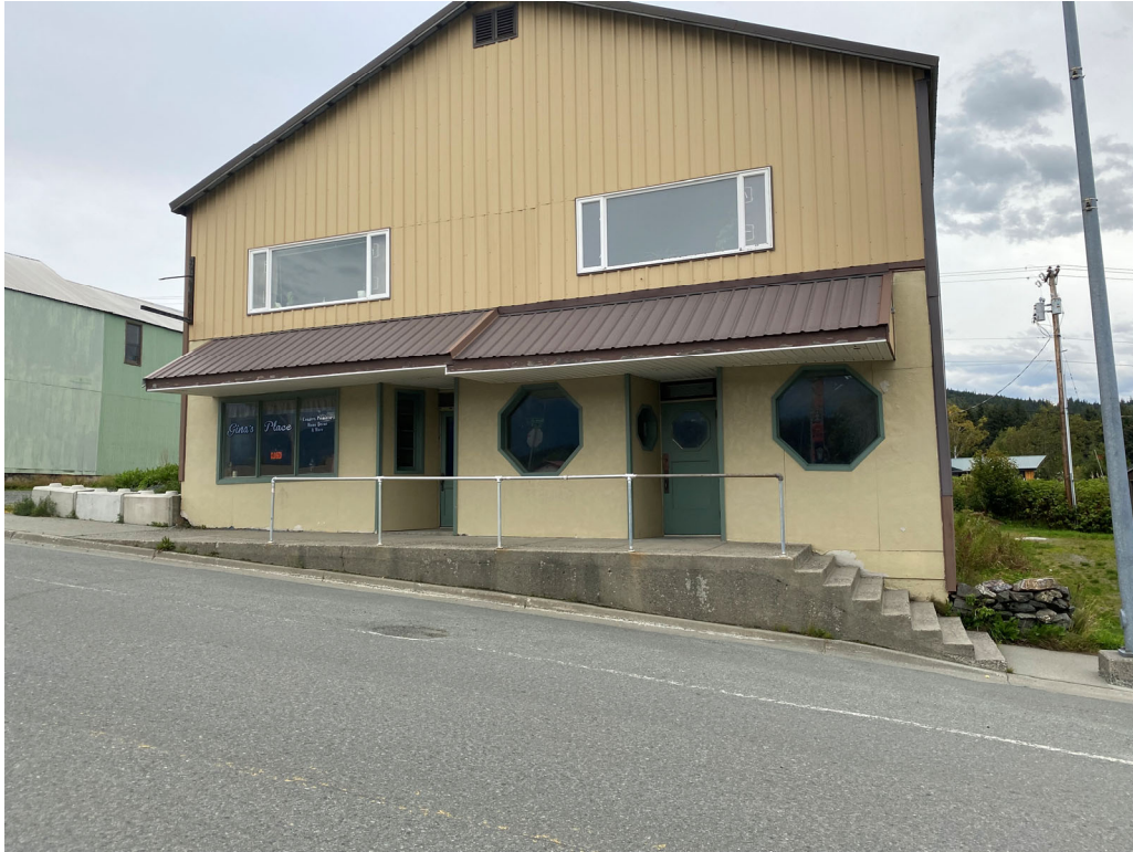
Figure 3 - Existing conditions at Pipe Hand Rail 2. Photograph dated 09/06/2022.
