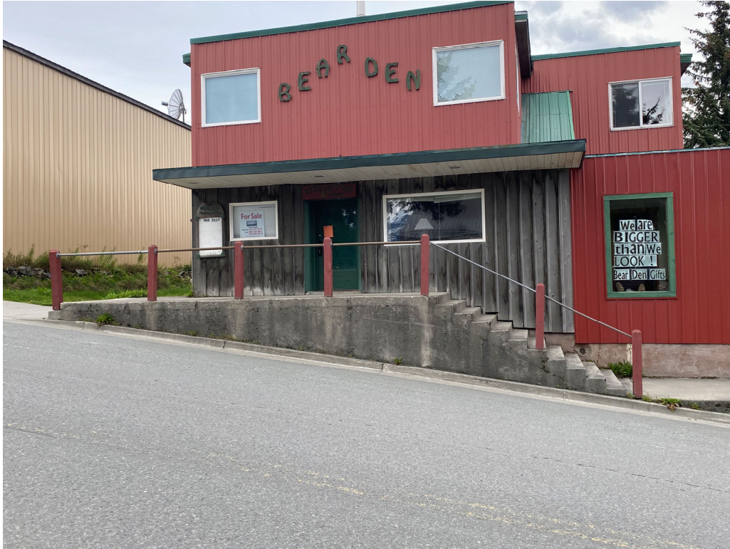
Figure 5 - Existing conditions at Pipe Hand Rail 3. Photograph dated 09/06/2022.
