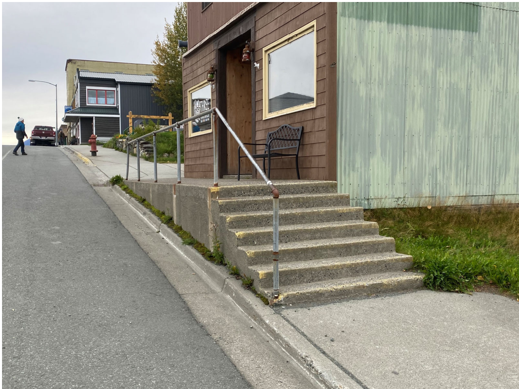
Figure 2 - Existing conditions at Pipe Hand Rail 1. Photograph dated 09/06/2022.
