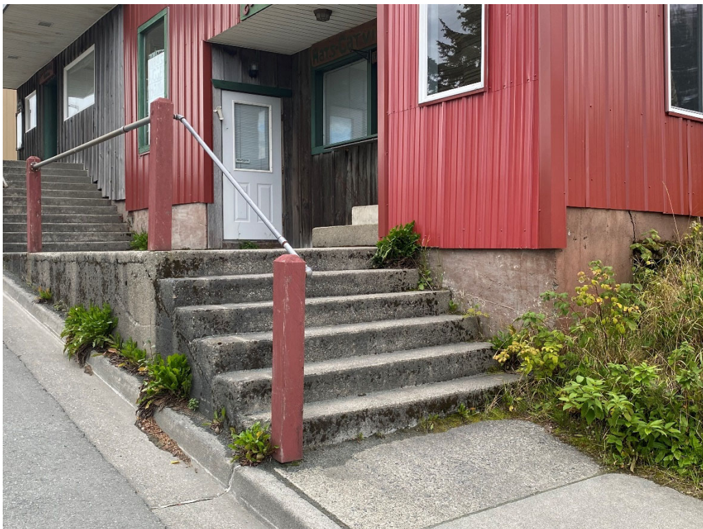
Figure 8 - Existing conditions at Pipe Hand Rail 3. Photograph dated 09/06/2022.
