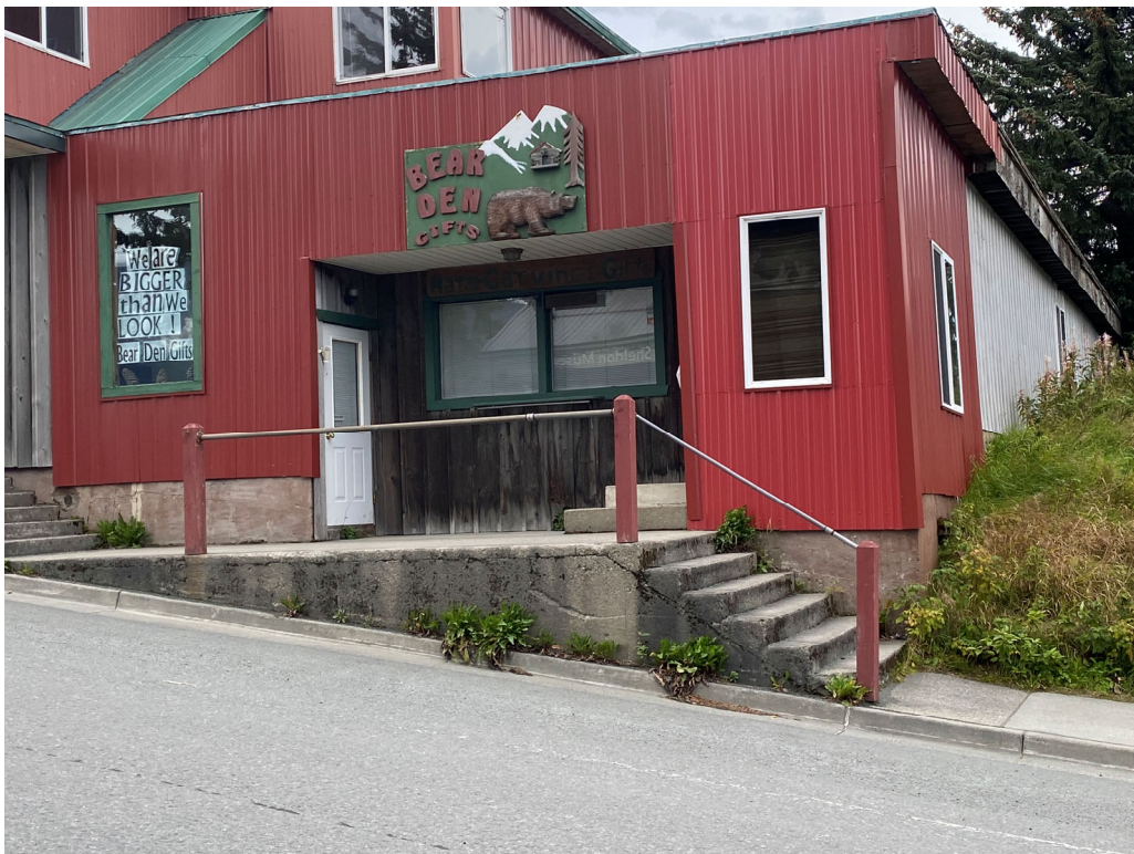
Figure 6 - Existing conditions at Pipe Hand Rail 3. Photograph dated 09/06/2022.
