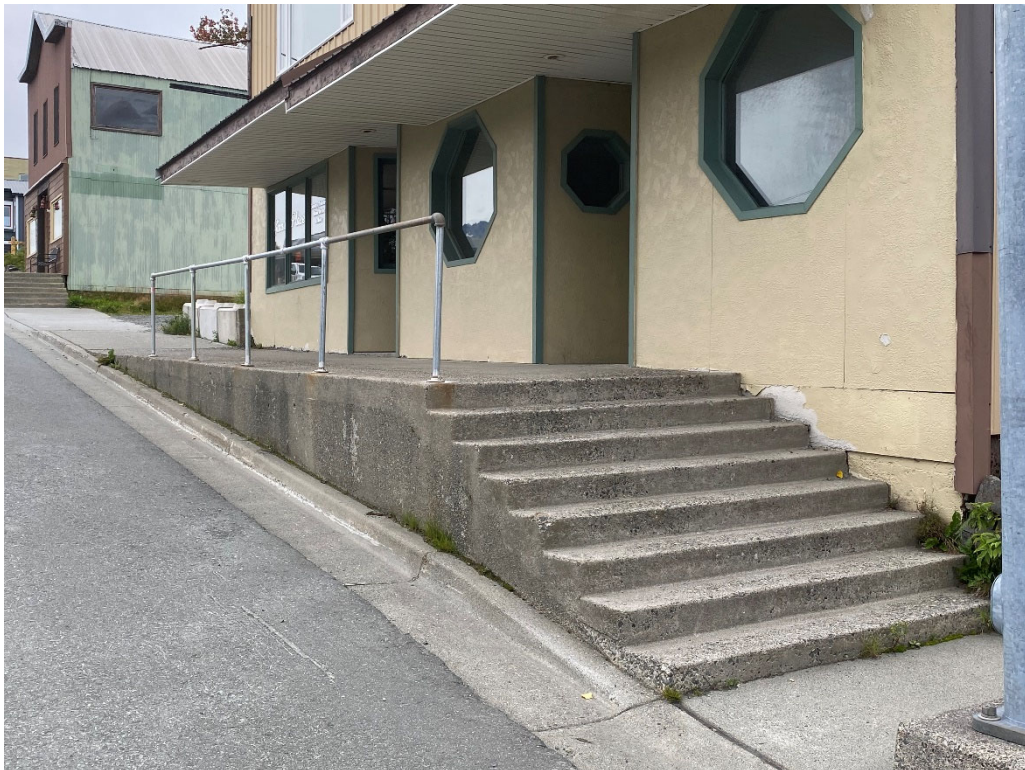
Figure 4 - Existing conditions at Pipe Hand Rail 2. Photograph dated 09/06/2022.
