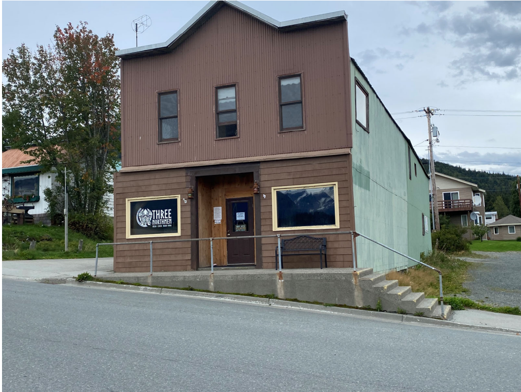
Figure 1 - Existing conditions at Pipe Hand Rail 1. Photograph dated 09/06/2022.
