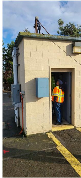
EXISTING WEATHERHEAD #2; TO BE REMOVED. REMOVE SUPPORT AND SEAL ROOF SURFACE WITH APPROVED PRODUCT.
