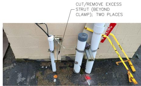
CUT/REMOVE EXCESS STRUT (BEYOND CLAMP); TWO PLACES
