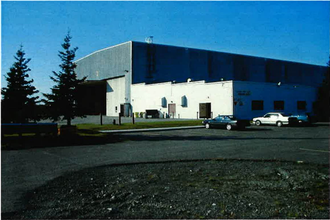
Photo 1. Hangar 6 in Anchorage, Alaska.
