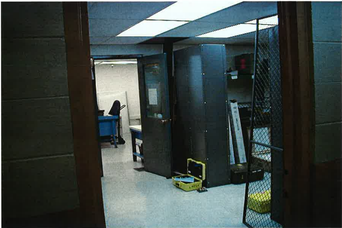
Photo 4. Hangar 6, 12- inch white vinyl floor tile and associated mastic.
