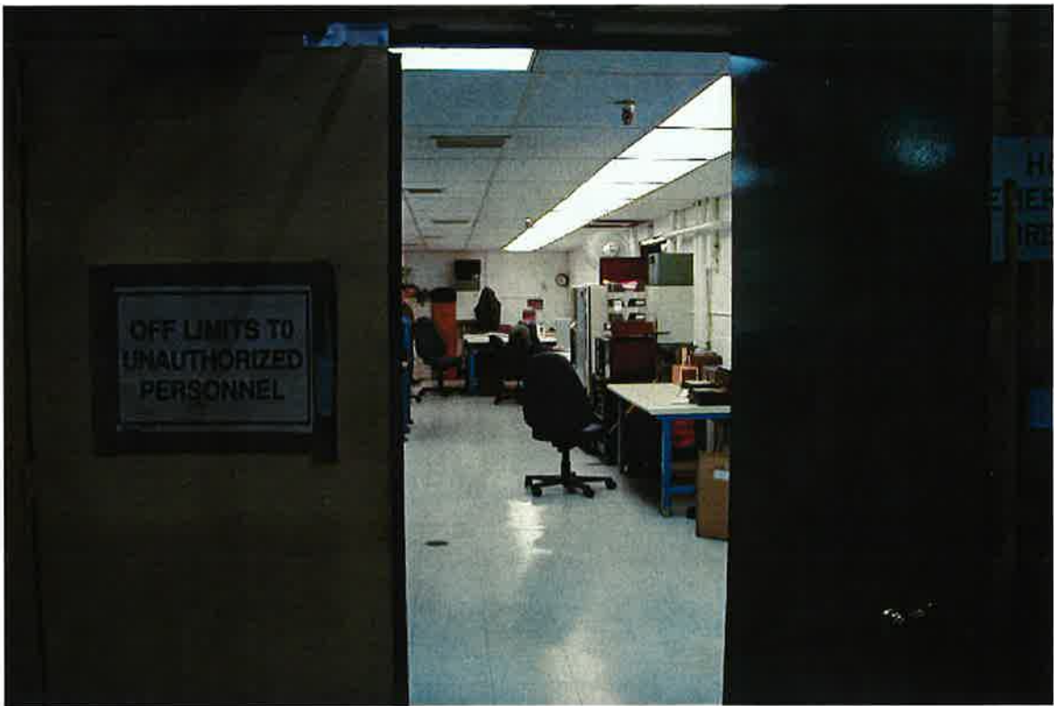
Photo 2. Hangar 6, 2- x 4- foot suspended ceiling tile.
