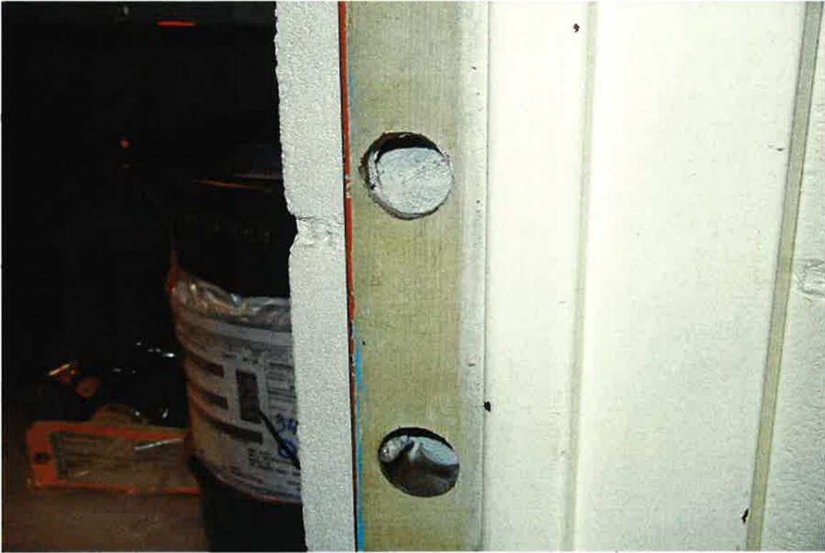
Photo 5. Hangar 6, Metal clad fire doors and frames.
