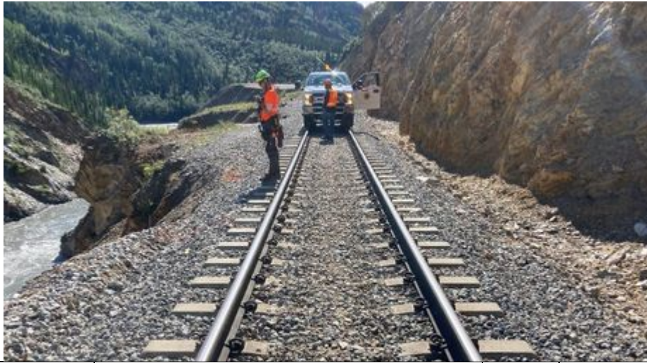
Comments: Center Point of Wall from Track Centerline Date: 7/28/2021
