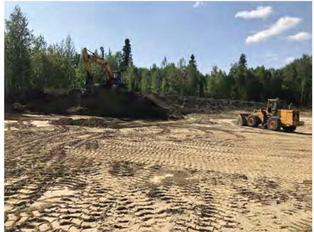
Photo 2: 20210804 Dismantling southern berm
