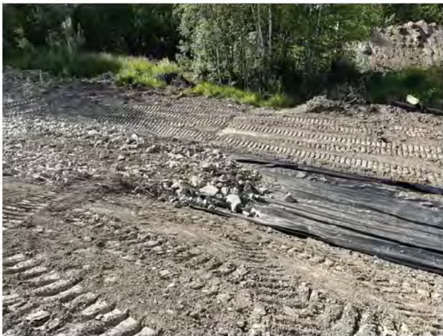
Photo 9: 20220723 Placing Riprap looking west
