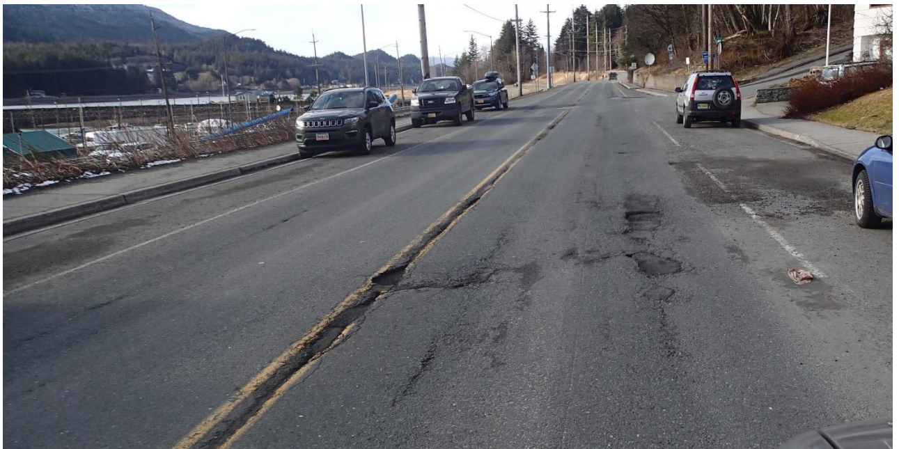
Figure 3: Same location as Figure 2, just South of Ross Way in Feb. 2020 shows significant deterioration including raveling and rutting.
