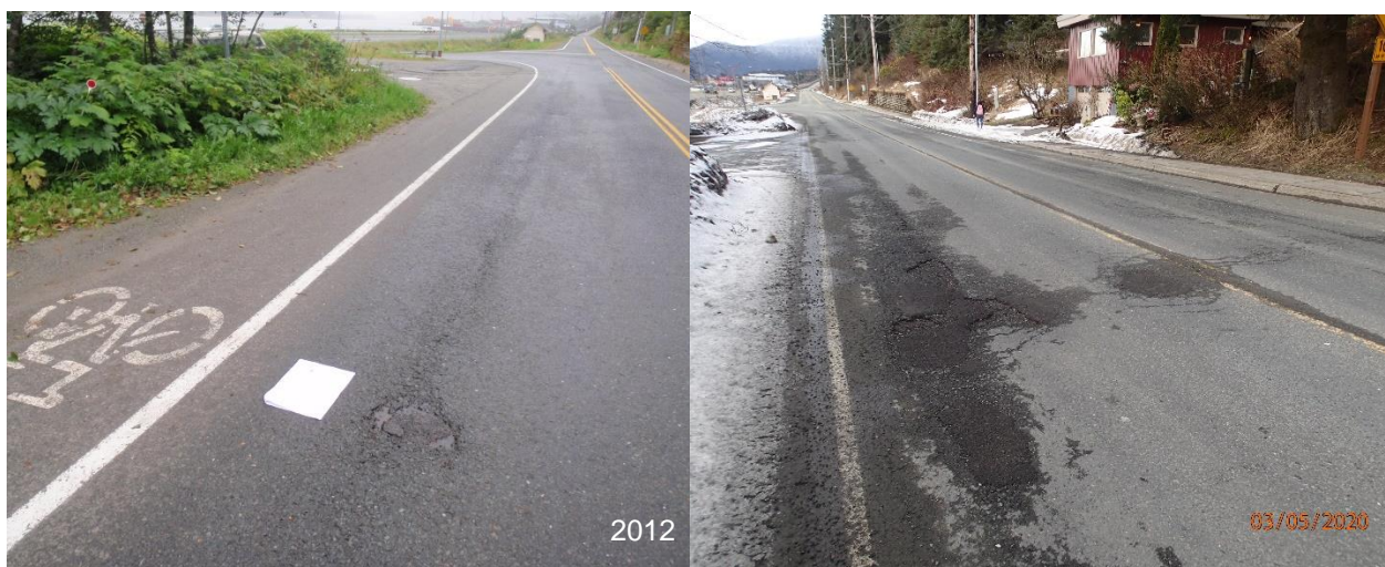
Figure 9: Continued deterioration and Heavy Cracking in the SB Lane at STA. 76+80.
