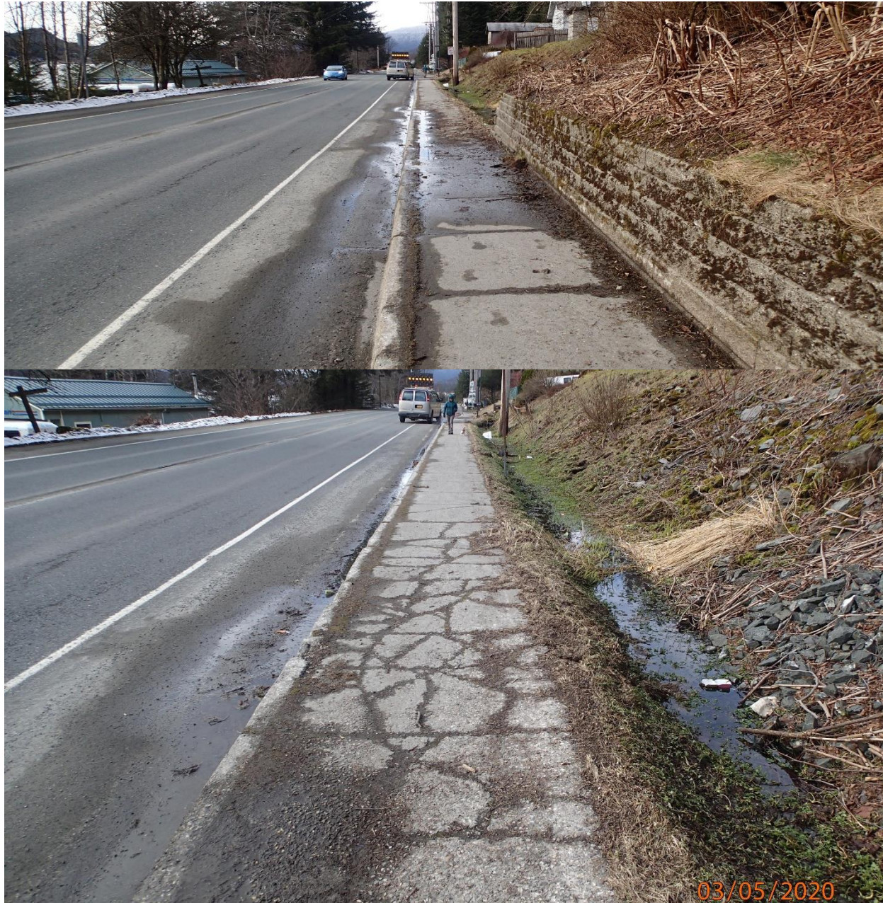
Figure 6: The sidewalk and Curb/Gutter at Sta. 59+00 and 59+75, has deteriorated significantly since 2012. It is possible this was caused from excavation efforts at the broken end of the retaining wall at that location. This location continues to “Weep” water from above.
