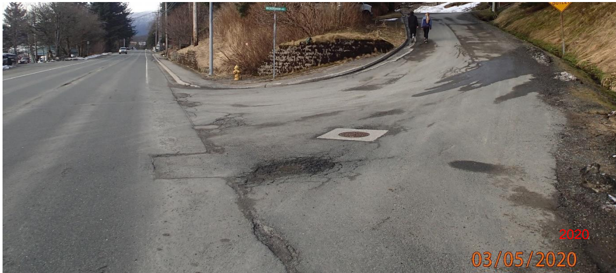
Figure 5-split: The continued deterioration of the intersection of Glacier Ave. and Wickersham Dr..
