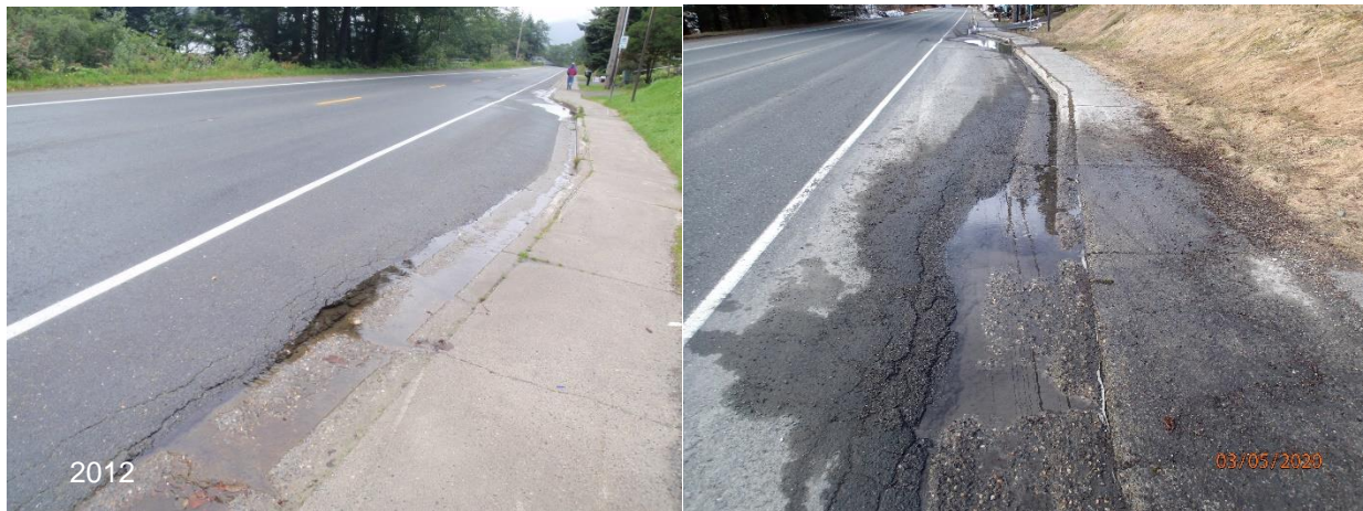
Figure 7: Continued deterioration and Heavy Cracking at the HDCP Ramp at the Bus stop STA. 61+50.
