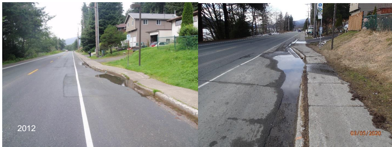
Figure 8: Continued deterioration and Heavy Cracking at the HDCP Ramp at the Bus stop STA. 62+10.
