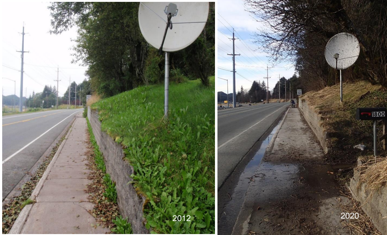
Figure 4: Typical retaining wall showing some leaning out at the top.
