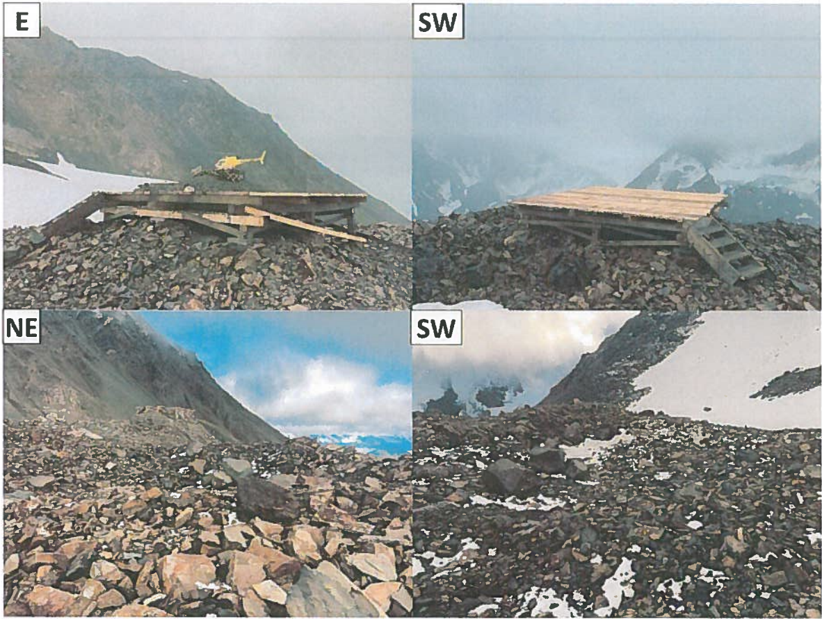
Photo 15: Paradise City Heli Pad unreclaimed (top) and reclaimed (bottom). Heli pad was both built and fully reclaimed in 2022.
