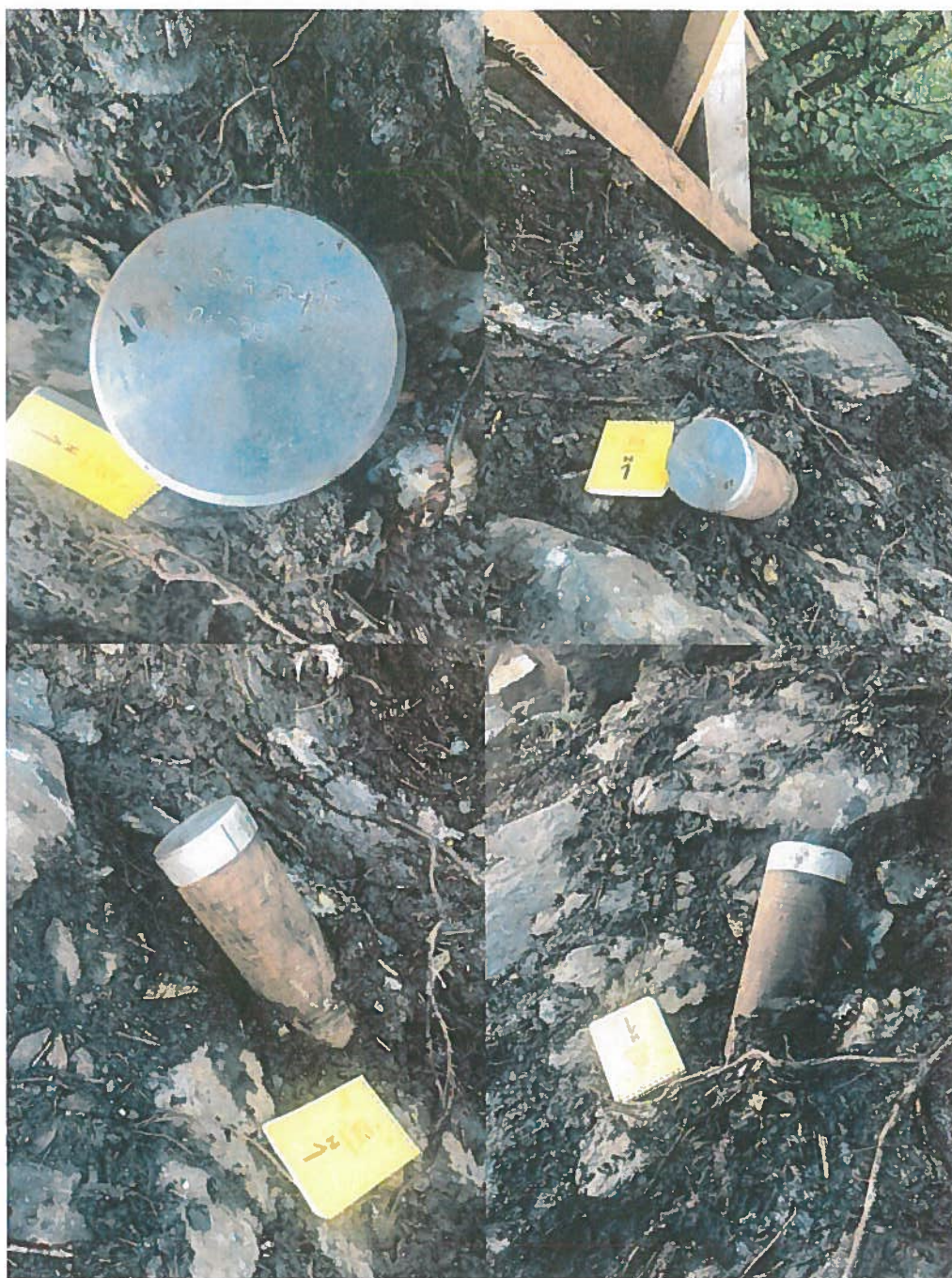
Photo 6: B-Lo Pad diamond drill hole CMR22-147 is capped. Mixed slotted and unslotted PVC was installed to support potential future geophysical surveys.
