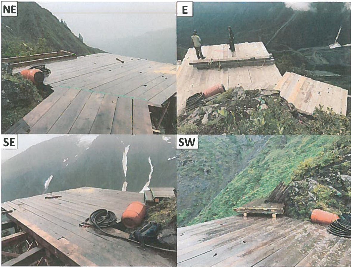
Photo 16: B-Lo Drill Pad pre-drill 2022, built in 2021.
