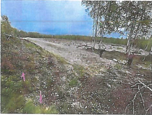
Photo 13: 20220824 looking NE complete
