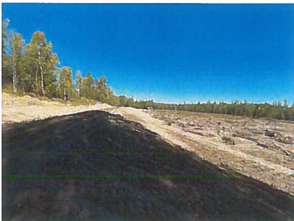
Photo 11: 20220811 northern portion looking east
