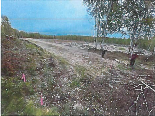
Photo 13: 20220824 looking NE complete
