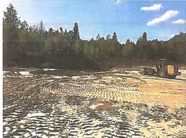
Photo 2: 20210804 Dismantling southern berm
