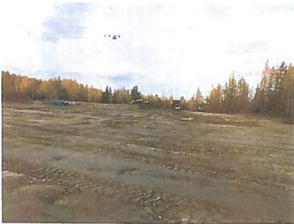
Photo 3: 20210921 Dismantling northern berm
