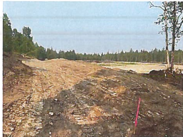
Photo 8: 20220630 Beginning of Diversion Ditch looking North
