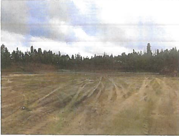
Photo 1: 20210728 Initial Lifts looking south
