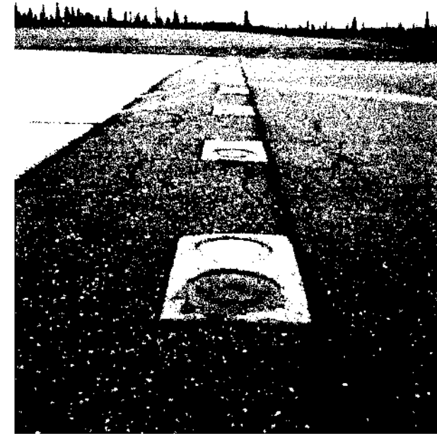
3 D2 DECOMMISSIONED R/W 29 THRESHOLD LIGHTS
