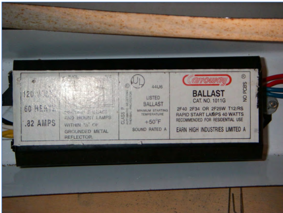
PHOTOGRAPH 10: FLUORESCENT LIGHT BALLAST IN LOFT.
