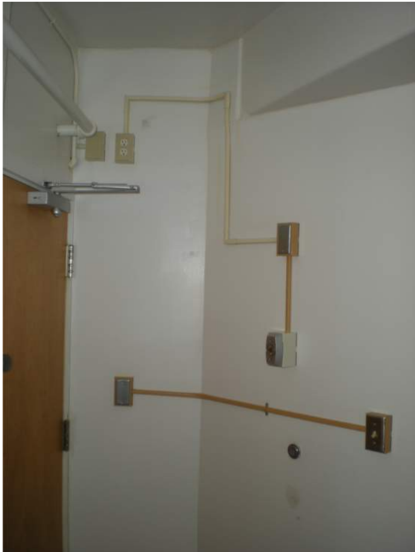
① PHOTO - ROOM 133
