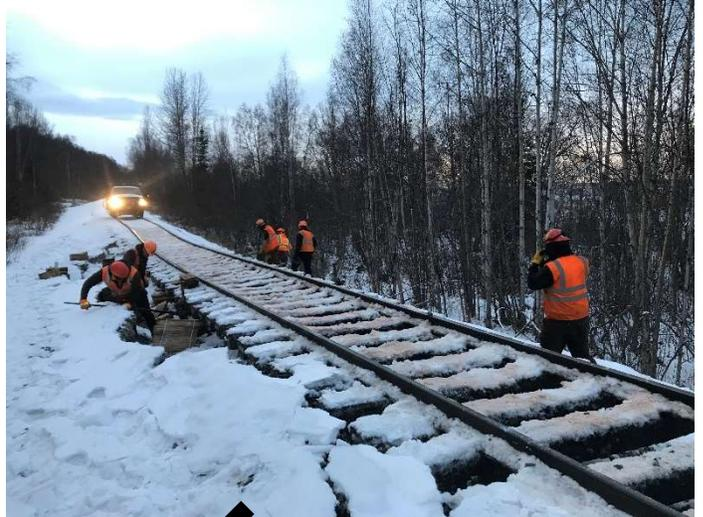
**Photo 2:** ARF & MOW forces jacking and shimming the affected section of rail at ≈MP 138.5, looking RR South-Southwest.
