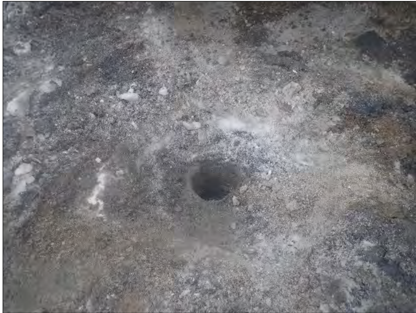
Photograph 26. Example of completed boring.
