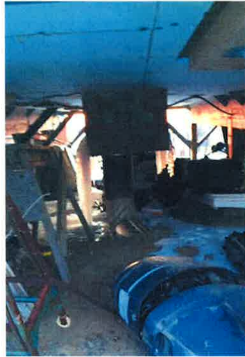
A water leak in an arctic box causing significant glaciation.
