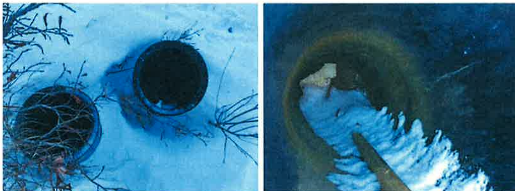
The water service shut off valves with covers removed and containing snow/debris.
