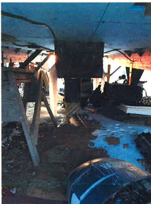
House 78 has a leak in the water arctic box that is glaciating on the sides of the box.
