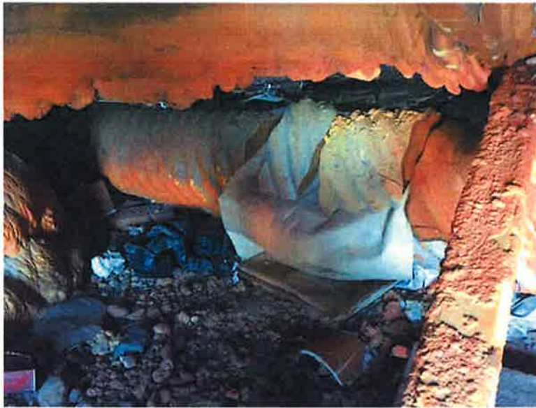
Building 159 sewer line that has been cut below the building.
