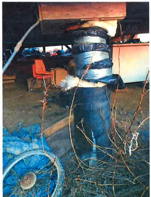
House 94. Water service line is being pulled out of alignment. Sewer line has pulled away from the arctic box and the owner has wrapped the ABS with insulation and plastic.
