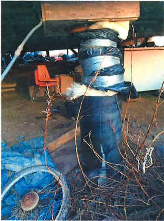
A homeowner repair to a service line that is pulling away from the arctic box.
