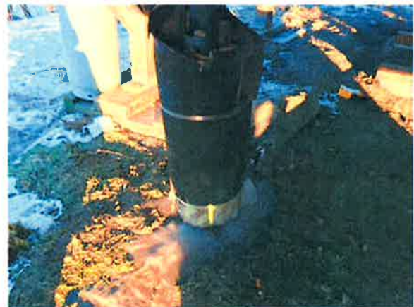
Sewer service separating from the arctic box. Glaciation also apparent on the ground.
