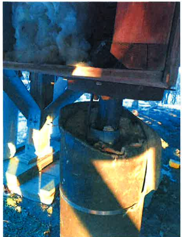
House 87. Water service line is being pulled apart at the 45joint where it enters the ground. Sewer line pulling away from arctic box and exposed ABS.
