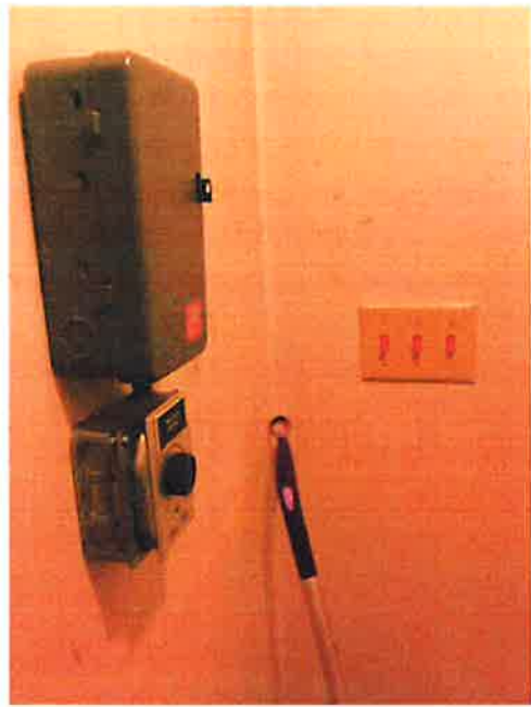
House 87. Water service entrance and heat trace switches (typical of all Phase 9 homes). No heat trace switches were labeled and most residents were unsure which were which.
