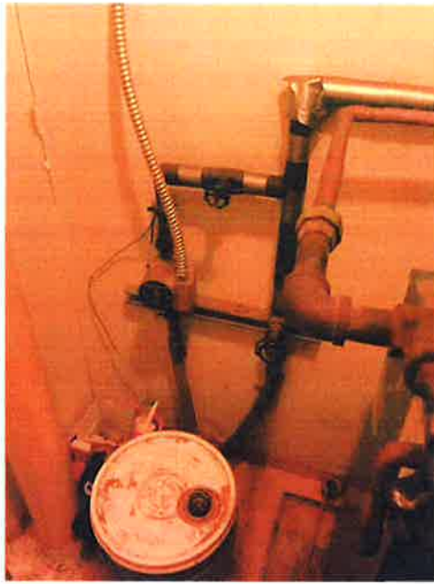
House 87. Water service entrance and heat trace switches (typical of all Phase 9 homes). No heat trace switches were labeled and most residents were unsure which were which.
