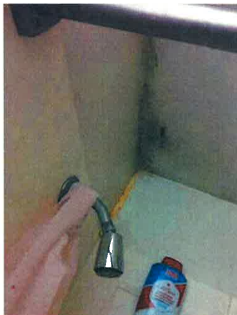
House 81. Mold in bathroom (typical of most Phase 9 homes) and Toyo water heater (typical of Phase 9 homes).
