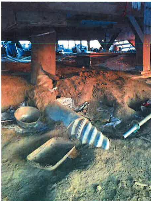
House 94. Water service line is being pulled out of alignment. Sewer line has pulled away from the arctic box and the owner has wrapped the ABS with insulation and plastic.
