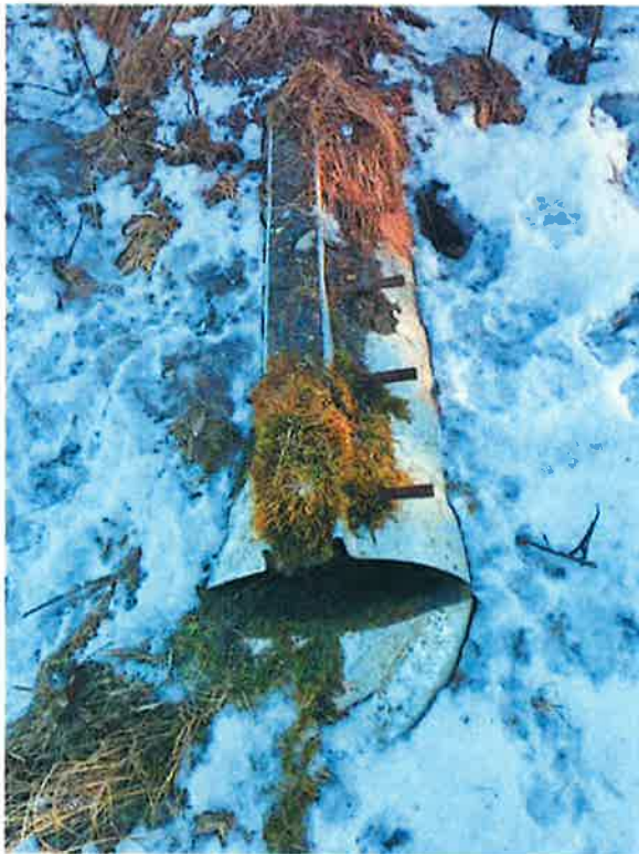
House 87. Water service line is being pulled apart at the 45joint where it enters the ground. Sewer line pulling away from arctic box and exposed ABS.
