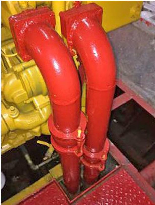
Figure 8.2C: Typical Cooler Piping at Generator, With Flexible Joint.
