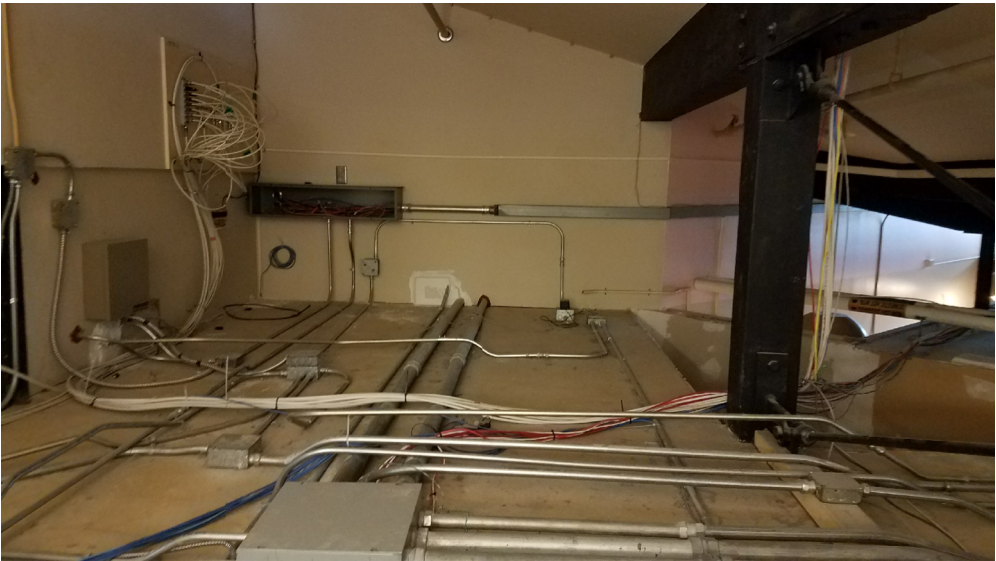
IMAGE 4: MECHANICAL MEZZANINE SURFACE MOUNT CONDUITS.
