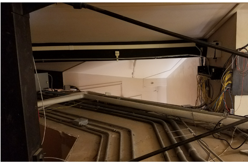
IMAGE 3: CONDUIT AND HYDRONIC PIPING AT PROPOSED WALL LOCATIONS.
