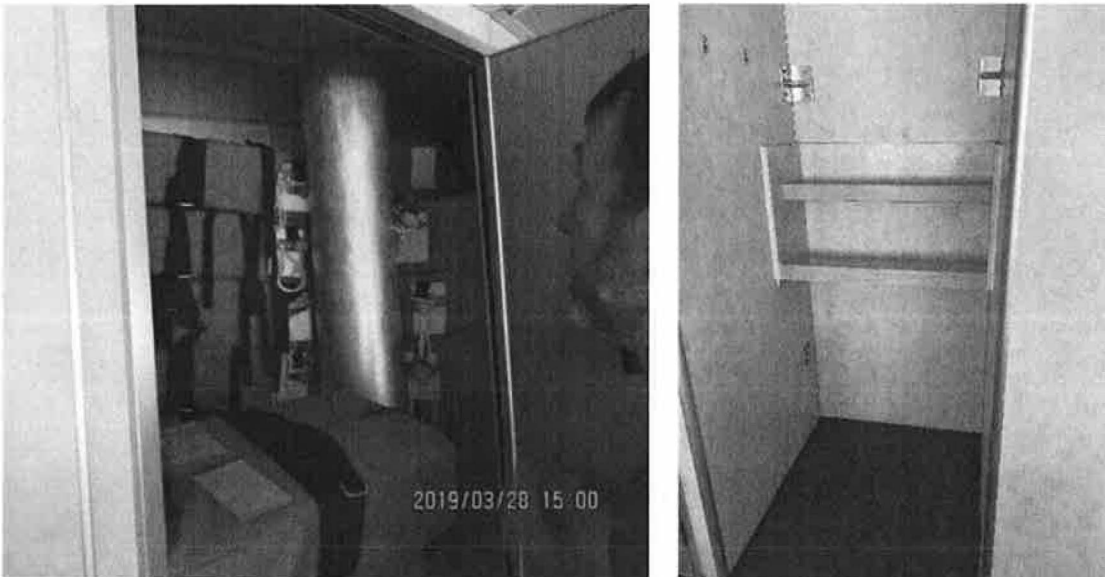
Figure 16 Lifejacket locker (left) and bracing from former phone booth (right)
