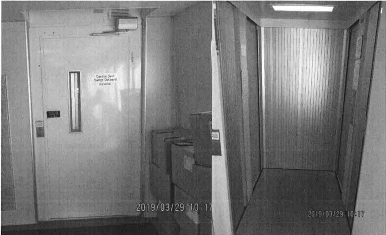
Figure 44 Passenger elevator on Passenger Deck
