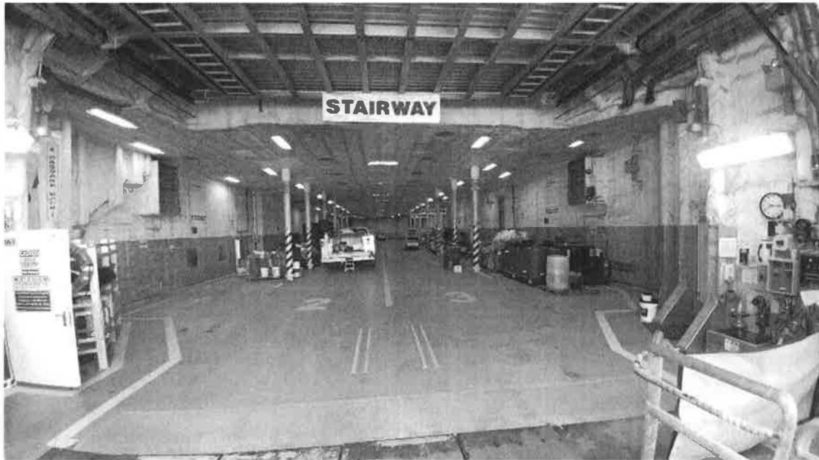
Figure 2 Vehicle deck view from stern door looking forward; insulation visible at sides and overhead
