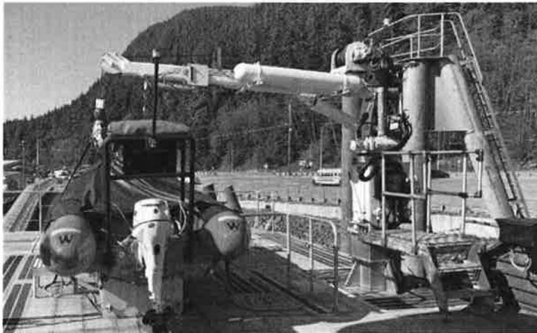
Figure 5 Rescue boat and davit on House Top
