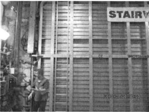
Figure 49 Vehicle Deck stern door and controls
