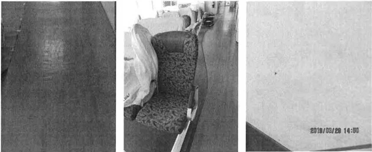
Figure 15 Bubbling in faux wood flooring (left), replacement seats (middle), and minor dents in bulkhead (right) in Forward Observation Lounge
