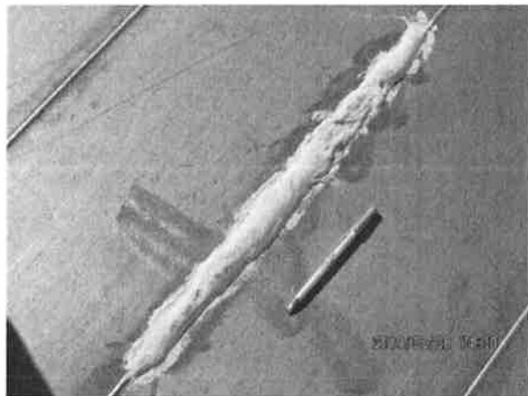
Figure 14 House Top (left) with caulking evident in many regions (right)
