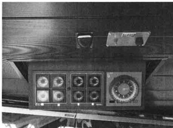
Figure 26 Waterjet steering system in Pilothouse on Bridge Deck
