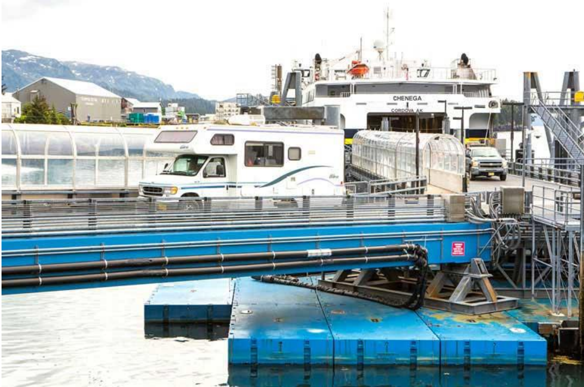
FVF Chenega Unloading Vehicles
