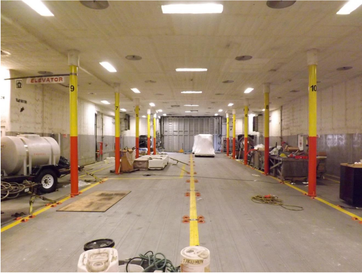
FVF Chenega Vehicle Deck Looking Aft
