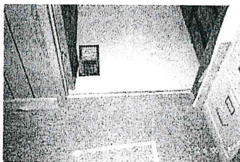
Photo No. 3 Shows painted plywood and carpet that are covering asbestos containing sheet vinyl.
