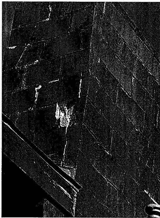
Photo 8: CMU Damage at Admin Building Chimney
