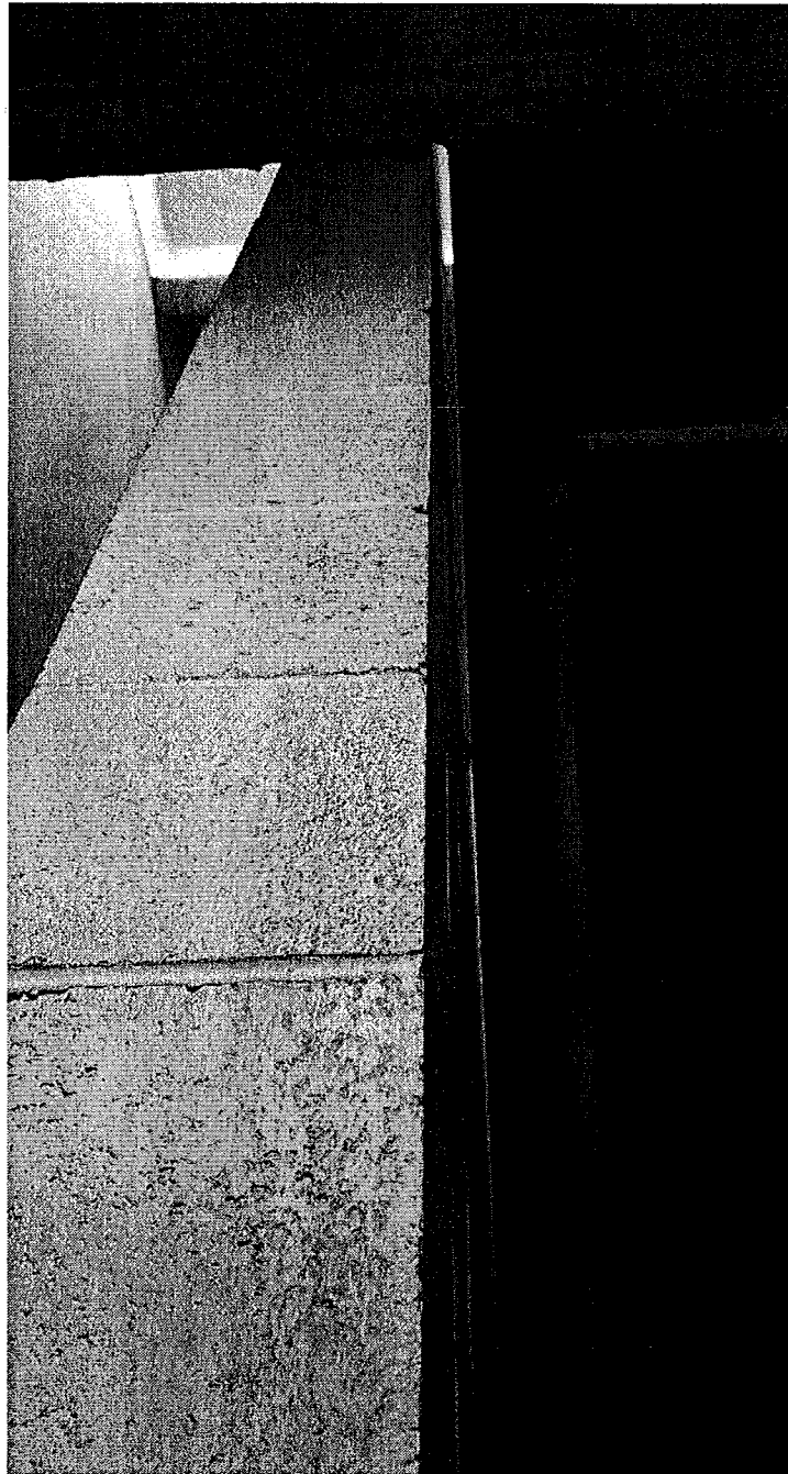
Figure 6 CMU Non-bearing Partition Wall in Stairwell: Separation as Seen From Underside of Wall
