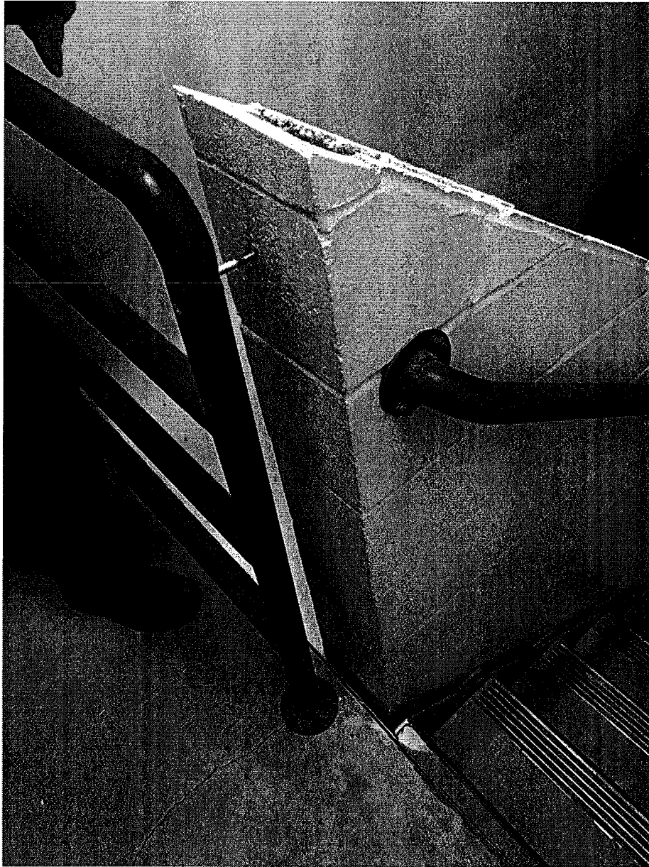
Figure 5 CMU Non-bearing Partition Wall in Stairwell: Separation as Seen From Top of Wall
