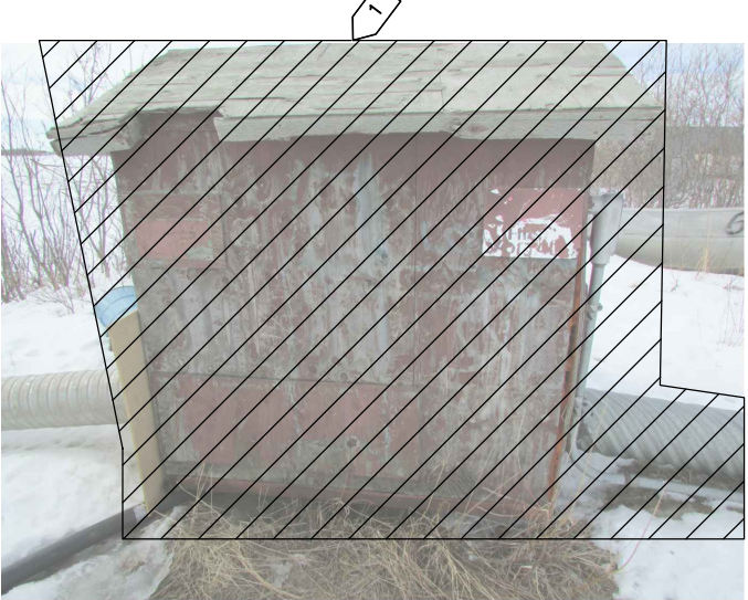
EXISTING RAW WATER PUMPHOUSE
