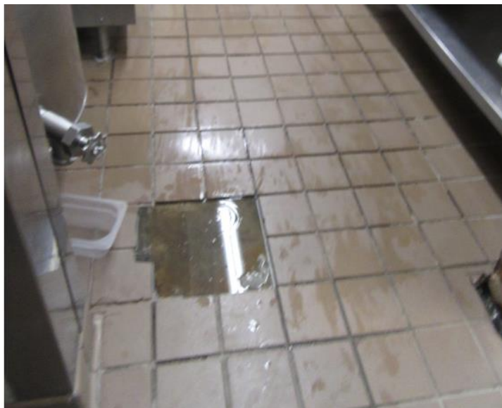
Picture 2- Kitchen Floor Damage
