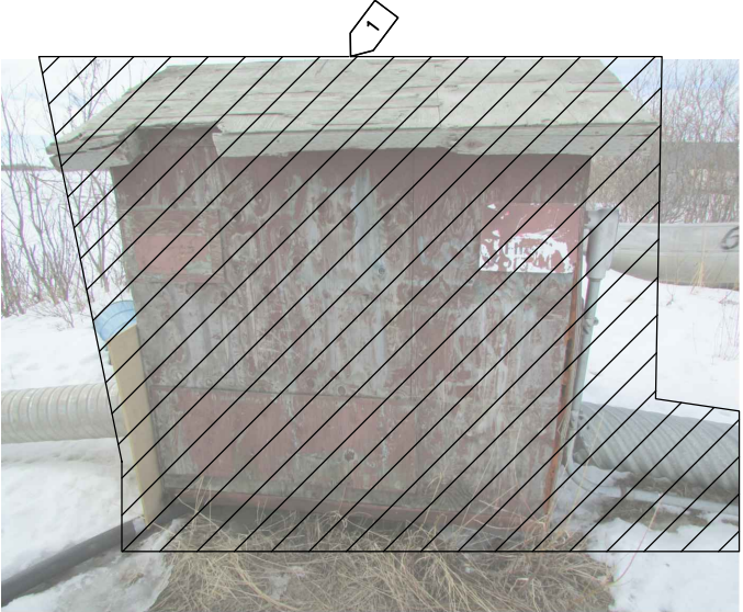
EXISTING RAW WATER PUMP HOUSE
