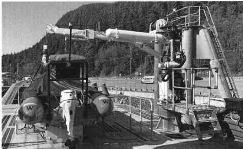
Figure 5 Rescue boat and davit on House Top
