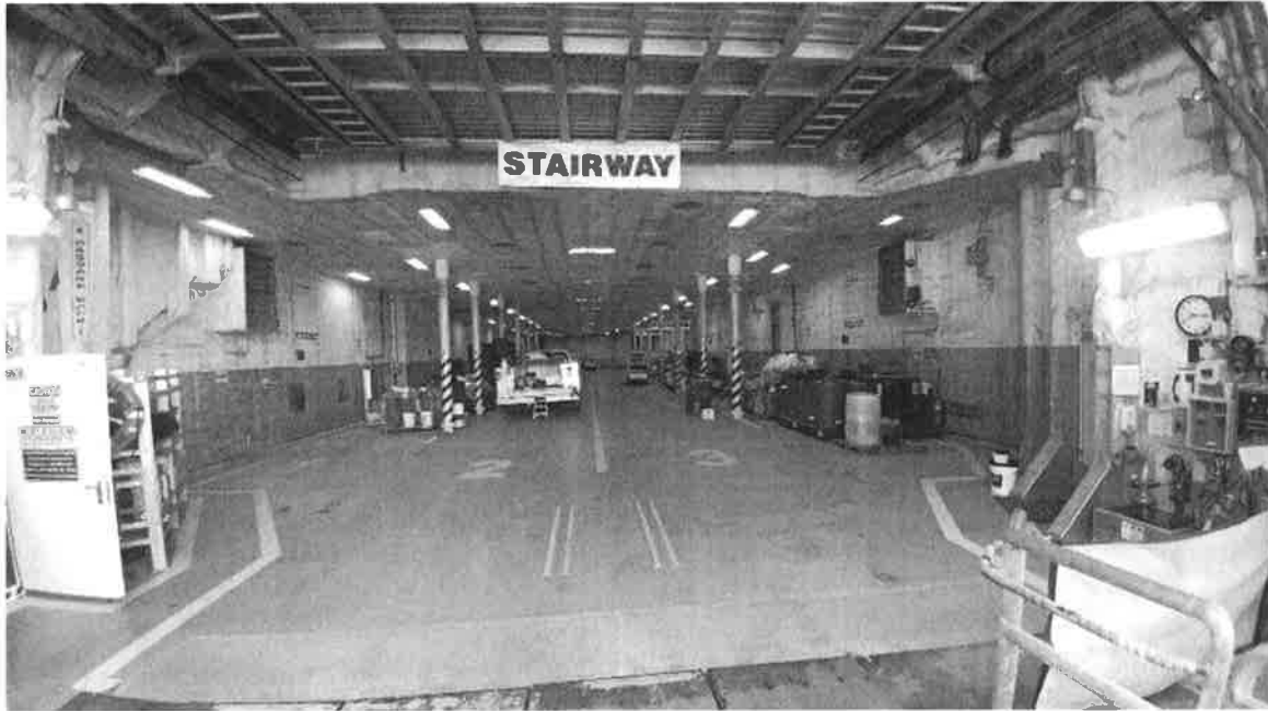
Figure 2 Vehicle deck view from stern door looking forward; insulation visible at sides and overhead
