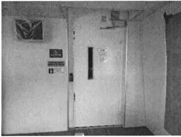
Figure 27 Passenger elevator on Passenger Deck
