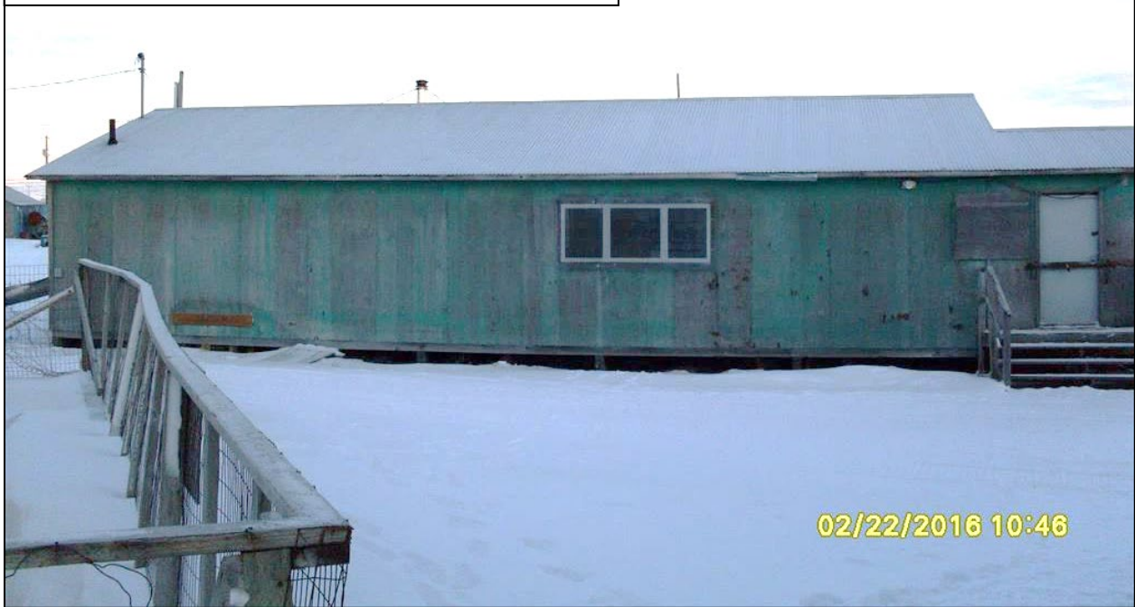
Boardwalk side of bldg., looking Northwest
