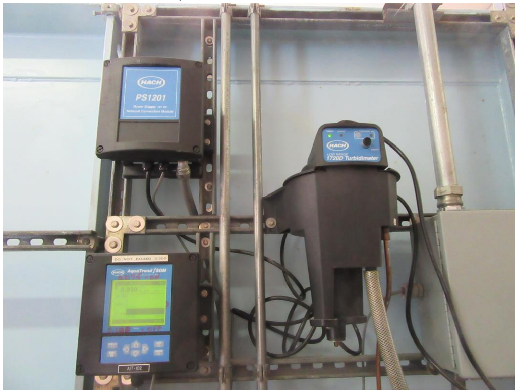
HACH 1720D turbidimeter, now obsolete:
