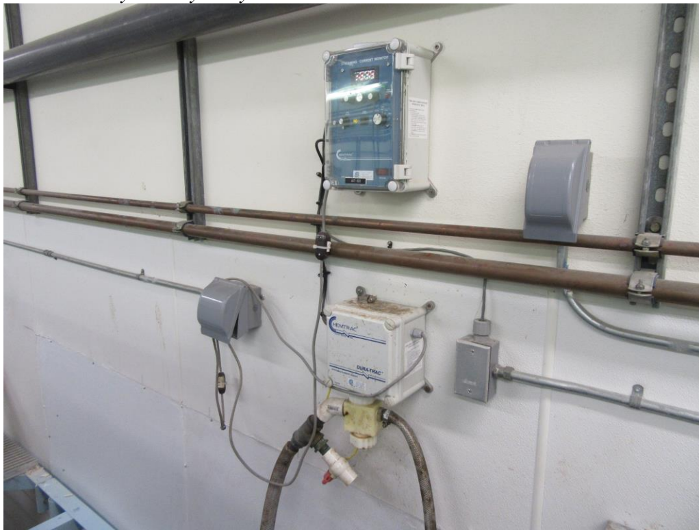
SCD assembly with hydrocyclone removed:
