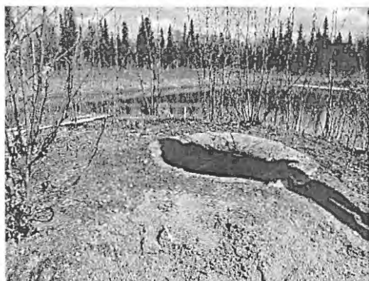
Manhole B, location of influent sampling
