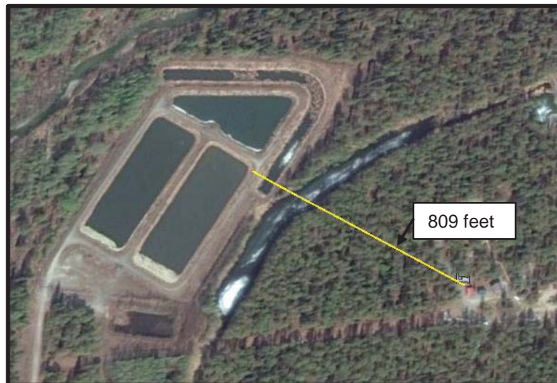
Figure 3: Separation Distance Between Existing Lagoon and Occupied Building
