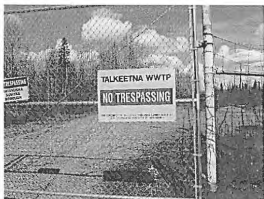
Signage posted at the lagoon gate fencing
