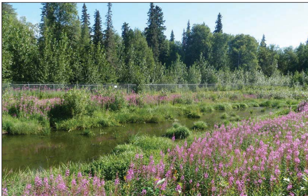
Figure 2-4: Talkeetna WWTF Constructed Wetlands from July 2016 Site Visit
