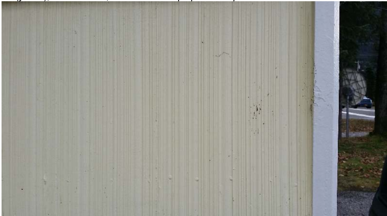
Photo 2: The yellow exterior paint had a lead concentration of 3.9 ppm, and the white trim had a lead concentration of 2.9.
