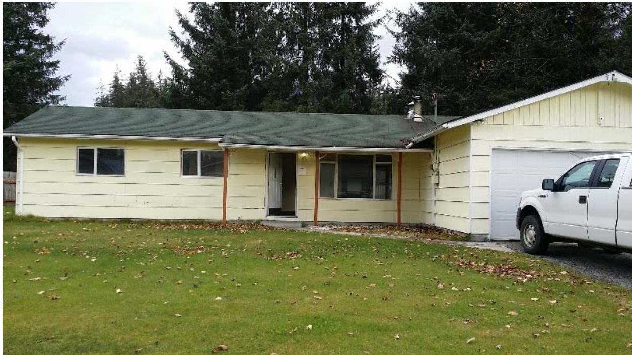
Photo 1: Lead-based paint was identified on the exterior of the house in the main exterior color (yellow), the white-trim, and a section of purple-brown paint.
