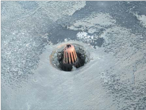
P5 - VIEW OF TYPICAL ROOF DRAIN
