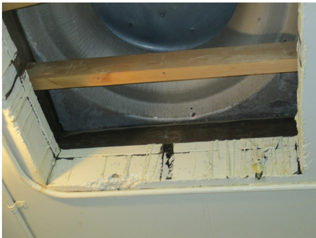
Photo 23: Wildwood Bldg 8 – Access Hole to Ventilator to be Framed-in
