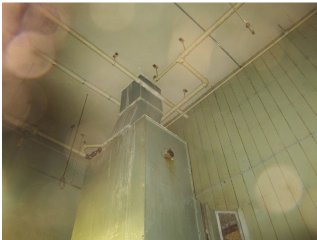
Photo 11: Wildwood Bldg 8 – Old Mechanical Duct Penetration to be Removed & Framed-in
