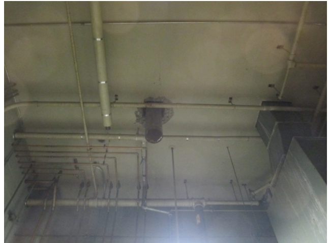
Photo 10: Wildwood Bldg 8 – Old Boiler Stack Penetration to be Removed & Framed-in
