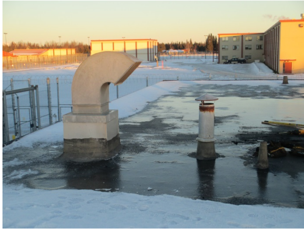
Photo 1: Wildwood Bldg 8 Main Roof - Mechanical Penetrations
