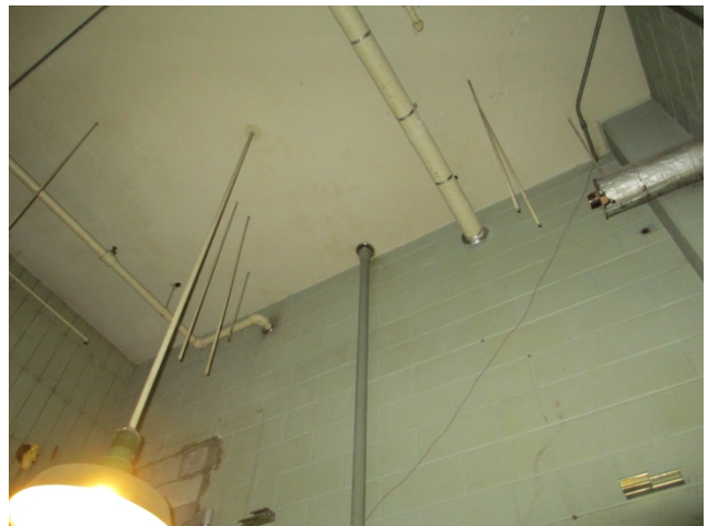
Photo 12: Wildwood Bldg 8 – Typical VTR Penetration to Remain (Sizes Vary)
