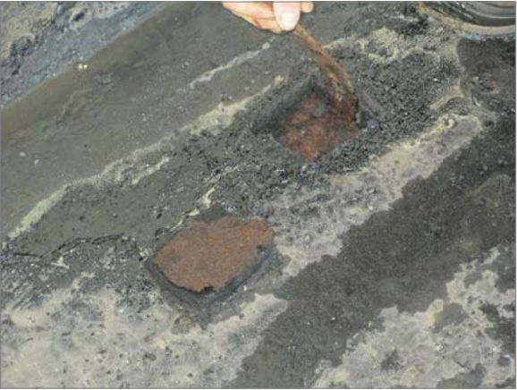
P11 - VIEW OF ROOF 'B' CORE CUT #2
