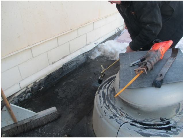
Photo 13: Wildwood Bldg 8 – Roof B @ Mechanical Room Core Cut #2 Prep w/ Ventilator to be Removed
