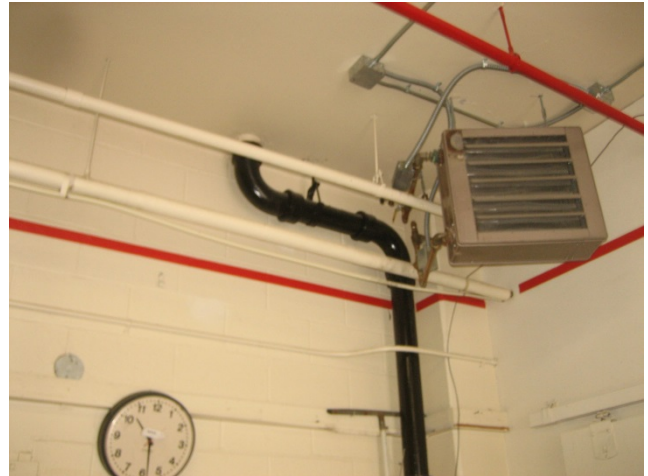
Photo 28: Wildwood Bldg 8 – View of Existing Roof Drain
