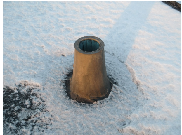
Photo 4: Wildwood Bldg 8 Main Roof - Typical VTR Penetration
