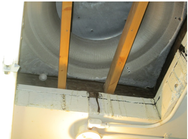
Photo 24: Wildwood Bldg 8 – Access Hole to Ventilator to be Framed-in
