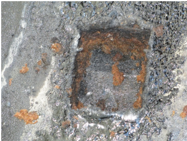
Photo 17: Wildwood Bldg 8 – Roof B @ Mechanical Room Core Cut #2 With Deck Exposed
