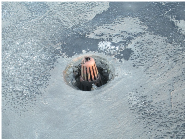
Photo 5: Wildwood Bldg 8 Main Roof - Typical Roof Drain
