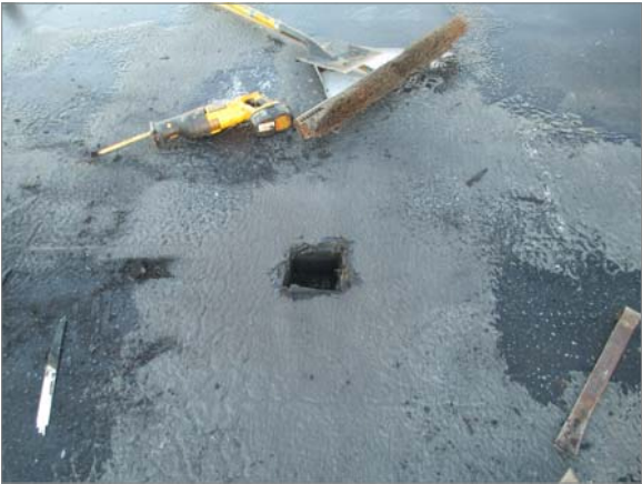
P4 - VIEW OF ROOF 'A' CORE CUT #1
