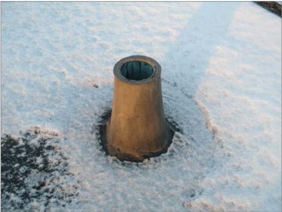
P6 - VIEW OF TYPICAL VTR W/ JACKET
