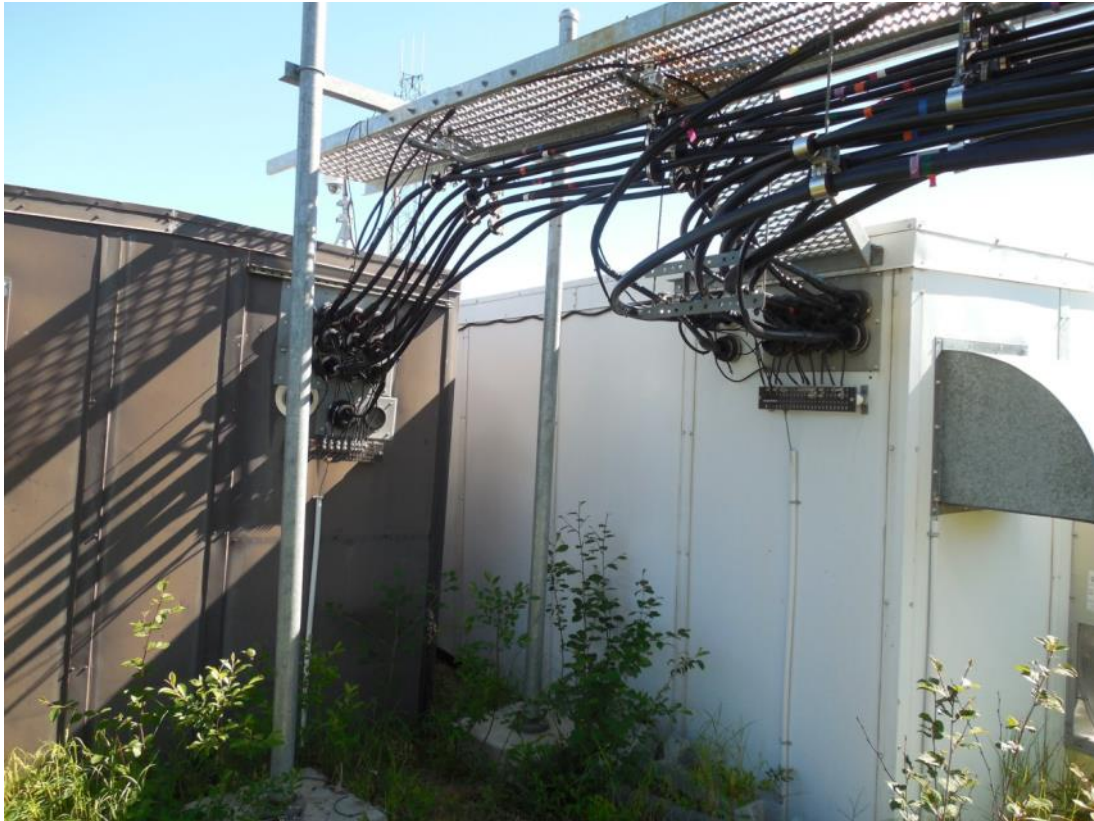
ESTER DOME – Ice bridge & entry ports
