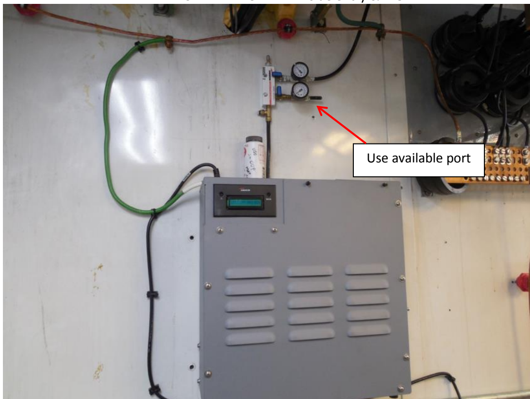
FAIRBANKS WATER TANK – Dehydrator & manifold
