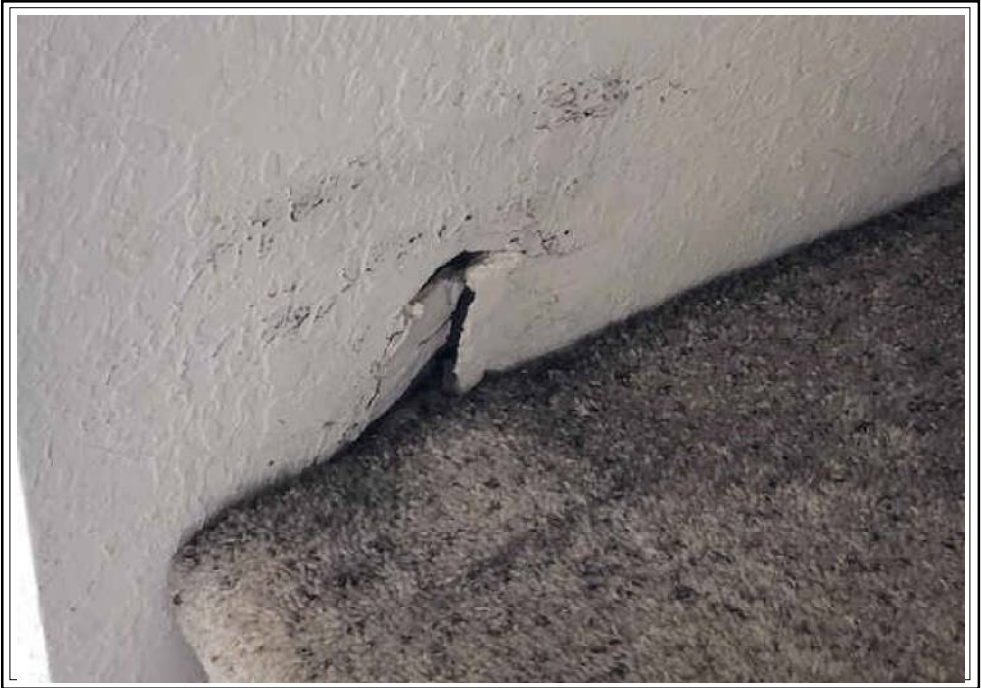
Some areas of damaged sheetrock.
