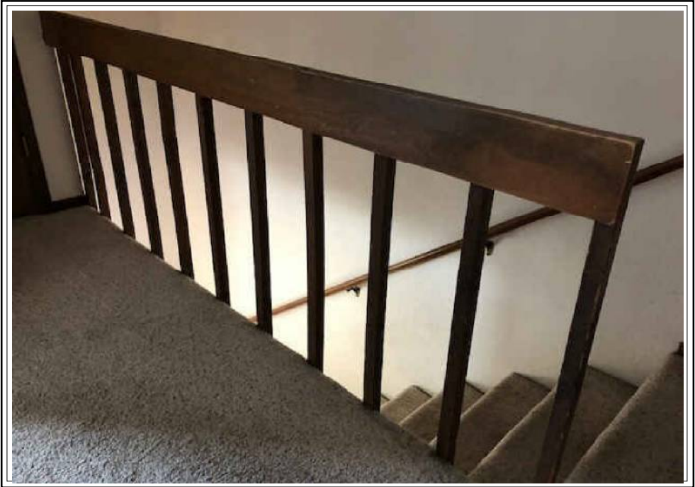
View of stair railings that do not meet current code for health or safety.
