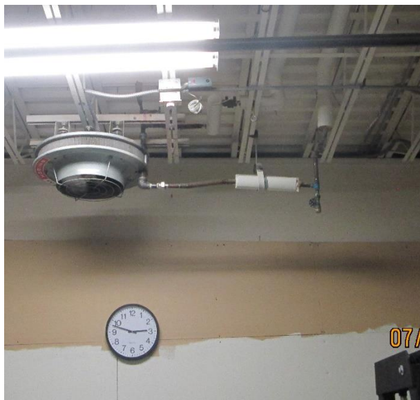
Partition wall showing gap at top of wall and mechanical/electrical equipment.
