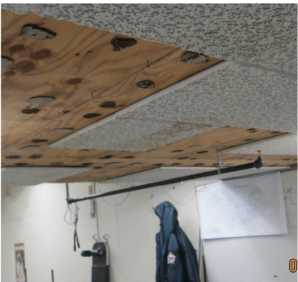
Close up view of sound proofing and adhesive on ceiling above fitness area.
