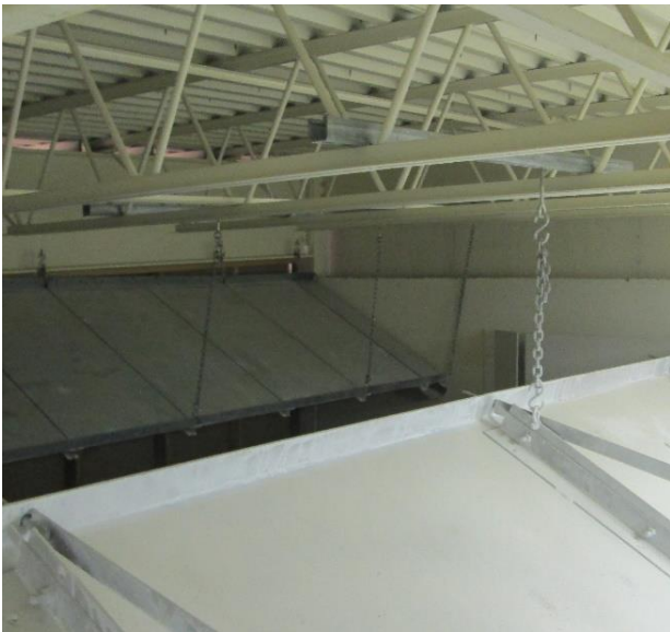
View above backstop showing baffle and partition wall with gap above.
